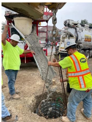
Contractor pouring concrete for the new traffic signal mast arm foundations
