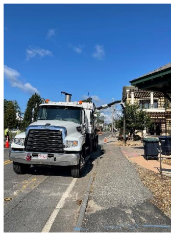
Large vacuum truck used to excavate for new traffic signal mast arm foundations. The deepest foundation was 12 feet deep!
