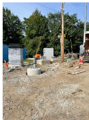
Finished concrete for traffic signal mast arms and controller cabinets.
