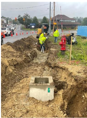
The contractor installing new conduit to support underground power for new decorative lighting
