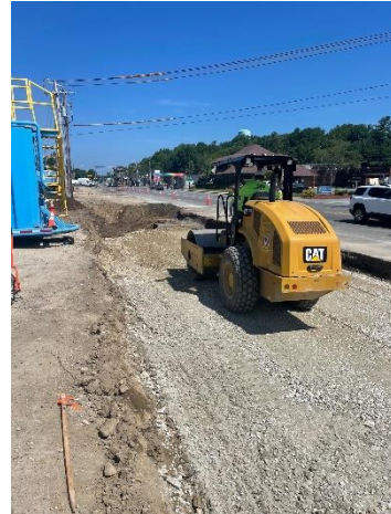
Contractor compacting newly installed road box widening base gravels.
