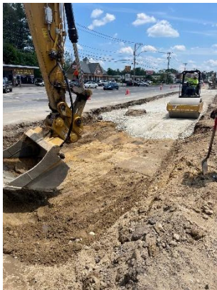
Road box widening on South Broadway near Salem Cooperative Bank.
