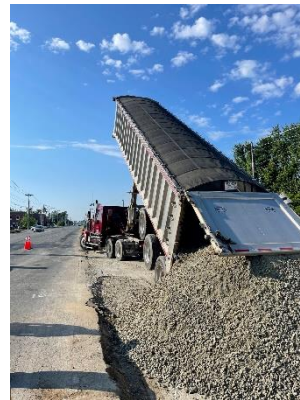
One of many deliveries of road base gravels needed to widen North and South Broadway.
