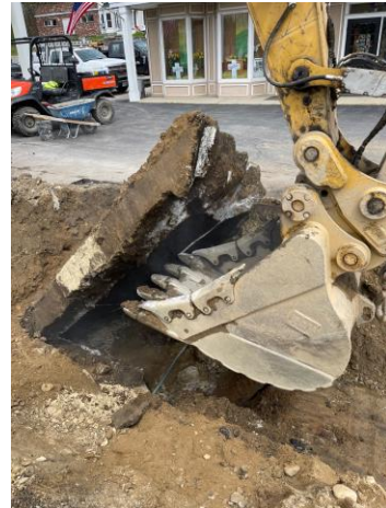
Removal of a cast in place concrete box culvert.
