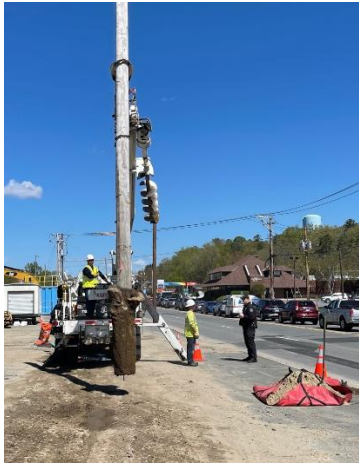
Removal of an existing utility pole.
