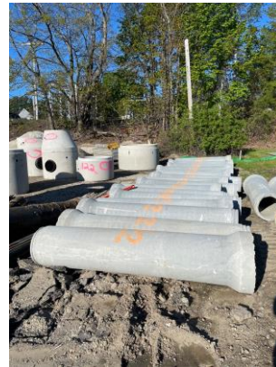
New reinforced concrete drain pipe being installed as part of the drainage upgrades.
