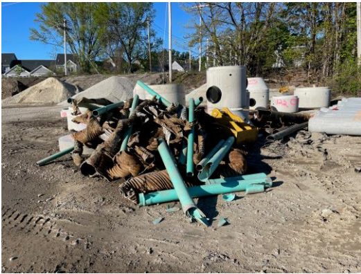
Pile of old corrugated metal drain pipe removed as part of the drainage upgrades.
