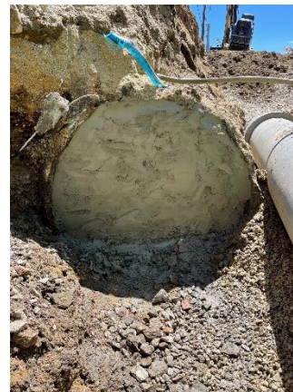
Brick and mortar bulkhead of an existing 36" diameter drain pipe to be abandoned.
