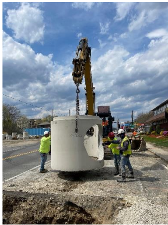
Installation of a large manhole adjacent to Salem Cooperative Bank.
