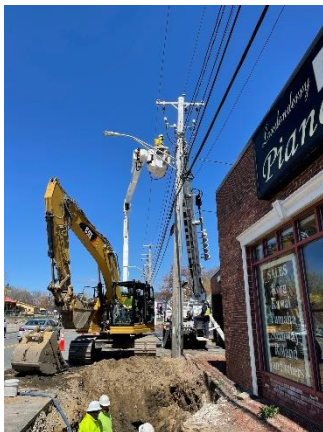
Liberty Utilities holding a utility pole adjacent to the drain pipe excavation to prevent the pole from moving.
