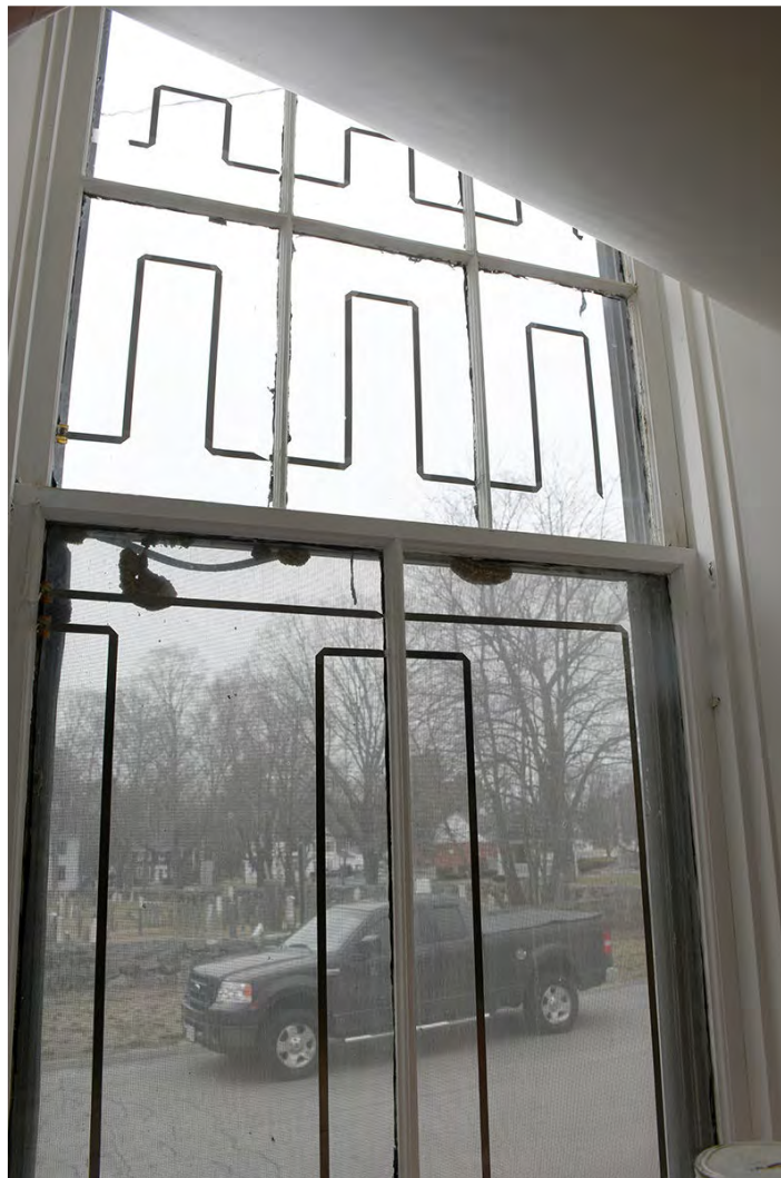
Photo 58: Window interior on south wall of first floor office. Electrical heat tape has been applied to the interior of each glass pane, and wasp nests are apparent on the exterior of the lower sash.
