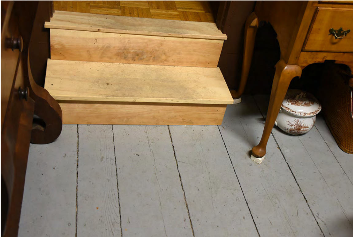
Photo 52: Painted pine flooring in the “bedroom” and the modern, elevated parquet flooring into the “kitchen” room.
