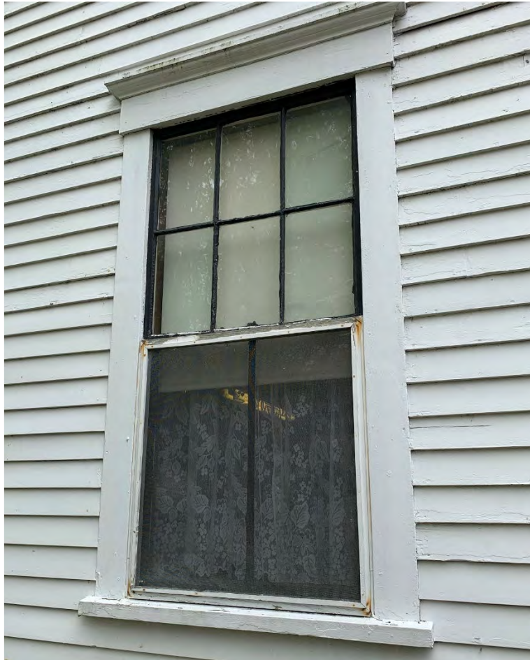
Photo 31: Window on the first floor, north elevation, with rusted screen installed over the lower sash.
