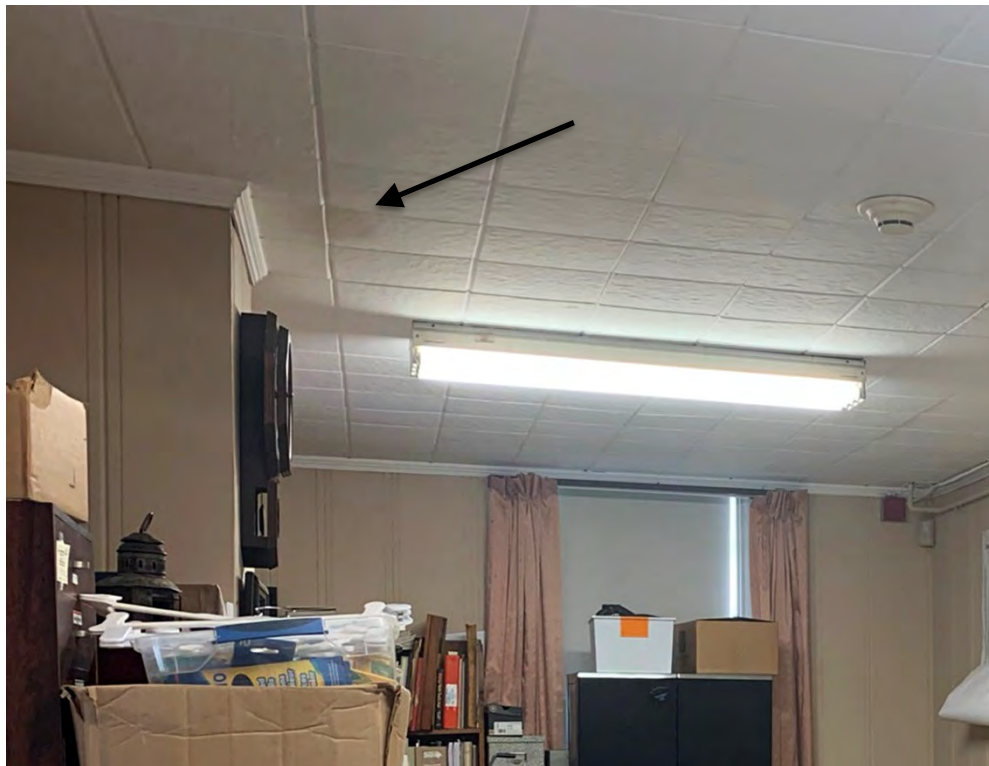
Photo 47: Small area of water staining in the ceiling tiles adjacent to the interior chimney stack.
