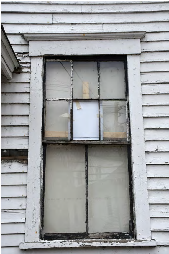
6/2 double-hung windows on the first-floor level.
