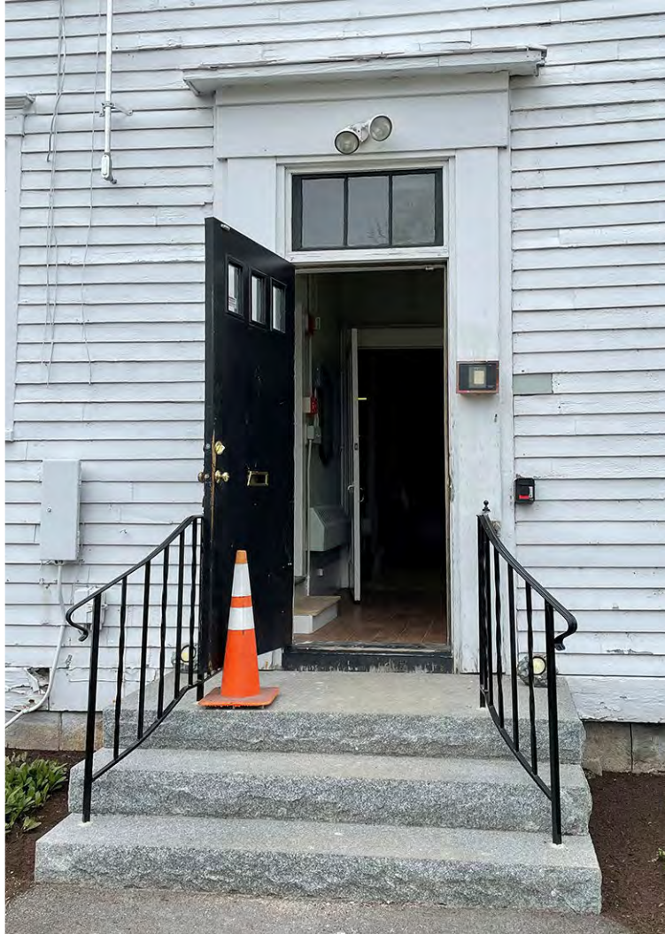
Photo 37: South elevation doorway. The current door is planned for replacement with a solid wood door. The granite steps are approximately 5-6 years old, and the metal railings were recently installed. The clapboards are in visibly poor condition on this side.
