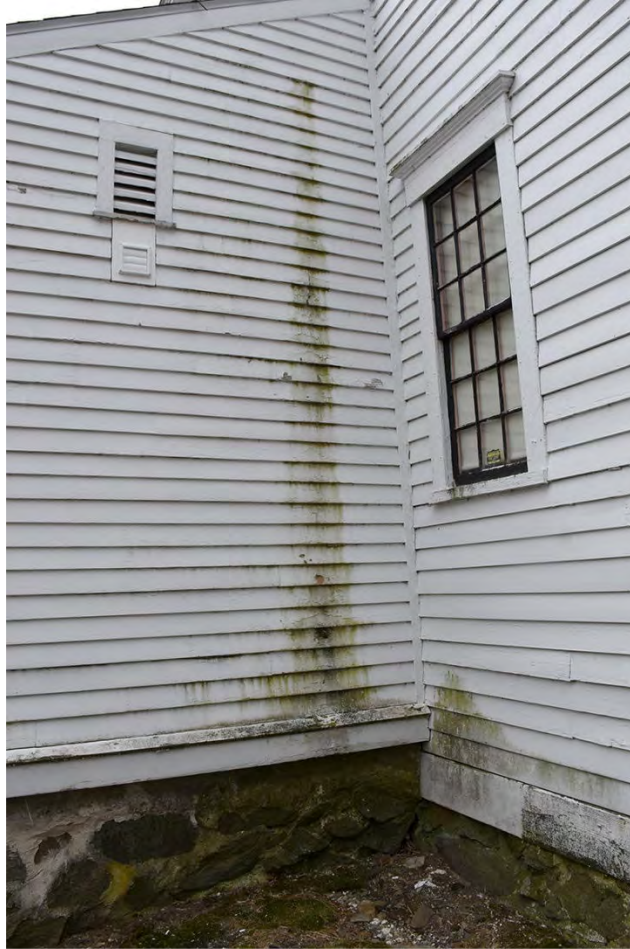
Photo 26: Biogrowth is seen on the clapboards and foundation walls in the north corner of the vault addition. The vents are for the area above the vault ceiling.
