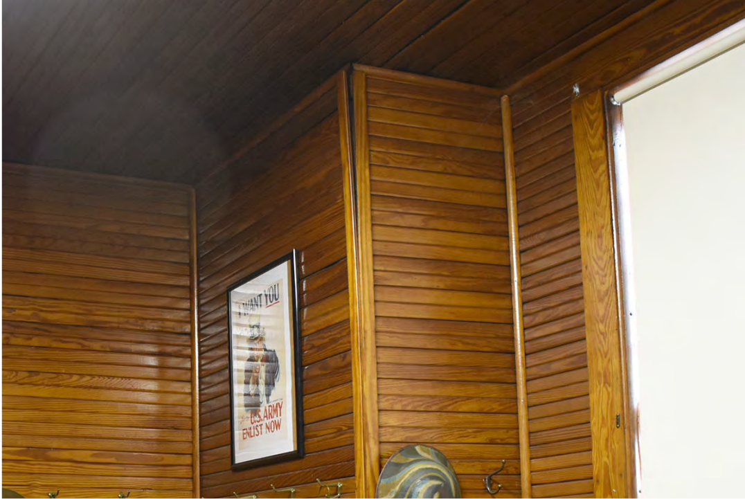
Photo 57: Chimney stack encased in beadboard in the "Military Room," edging strips are pulling away at the top corner.
