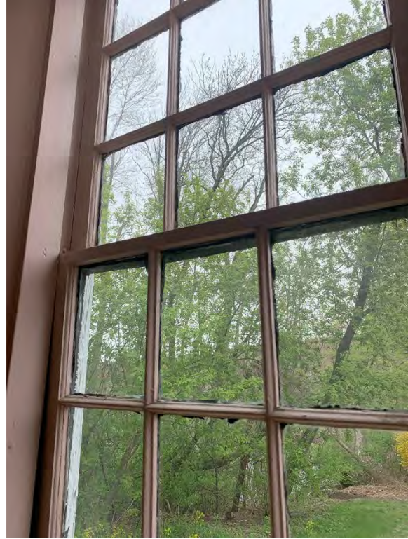
Window interior of 9/9 window on east wall in kitchen Photo 61: (left) and in the main room Photo 62: (right). Muntins have severe deterioration, and upper and lower sash do not meet properly. Window muntins differ, showing the use of sash from different time periods.
