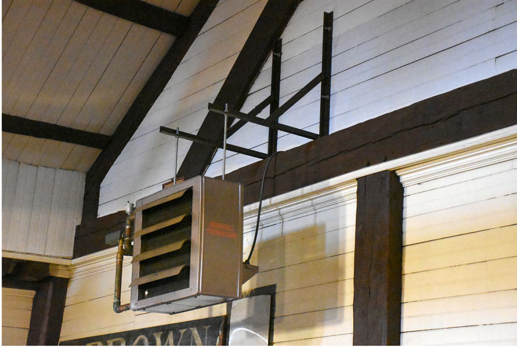
Photo 70: One of two heating units mounted on the north wall of the second-floor hall.
