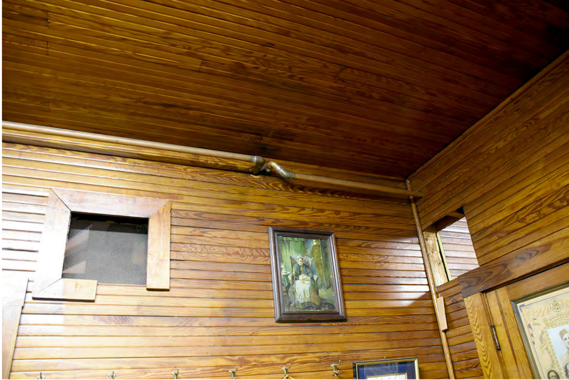
Photo 56: Openings have been cut into the upper walls of the “Military Room” for ventilation.
