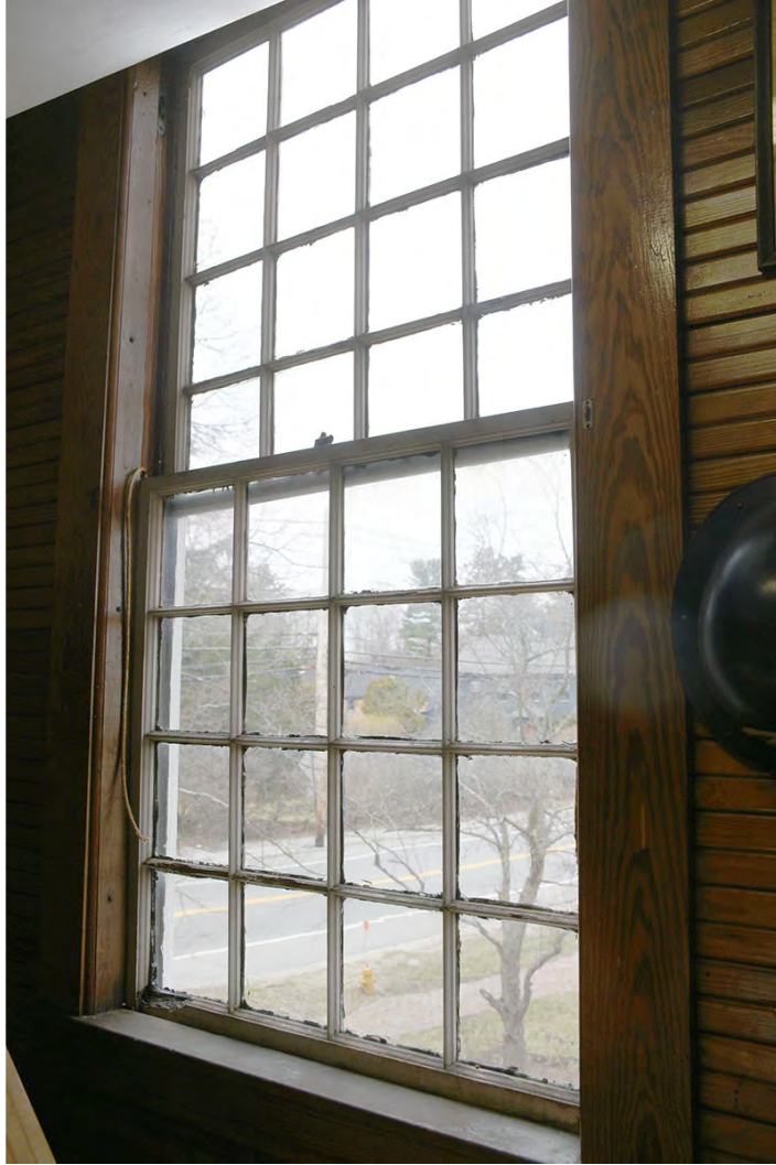
Photo 60: Interior of the north window in the “Military Room” showing a broken sash cord and rot/deterioration of the muntins and lower rail of the lower sash. This is one of the few windows with sash weights and cords.
