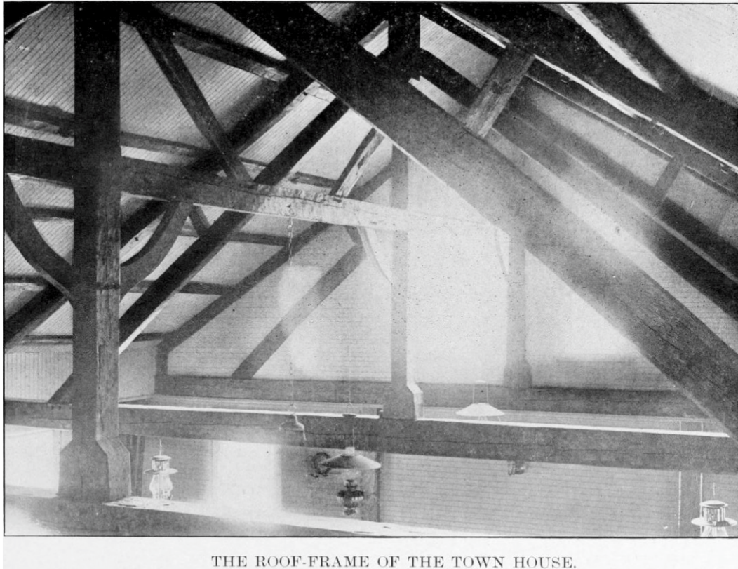
Figure 6: Searles's 1900 renovation highlighted the 1738 roof framing of the building, adding paired windows. This view is of the north wall, onto which an addition was built in 1908. (Gilbert 1907: 81)
