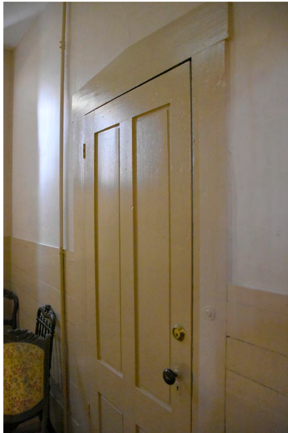
Photo 22: Door with peaked header at second floor stair hall, in southeast corner
