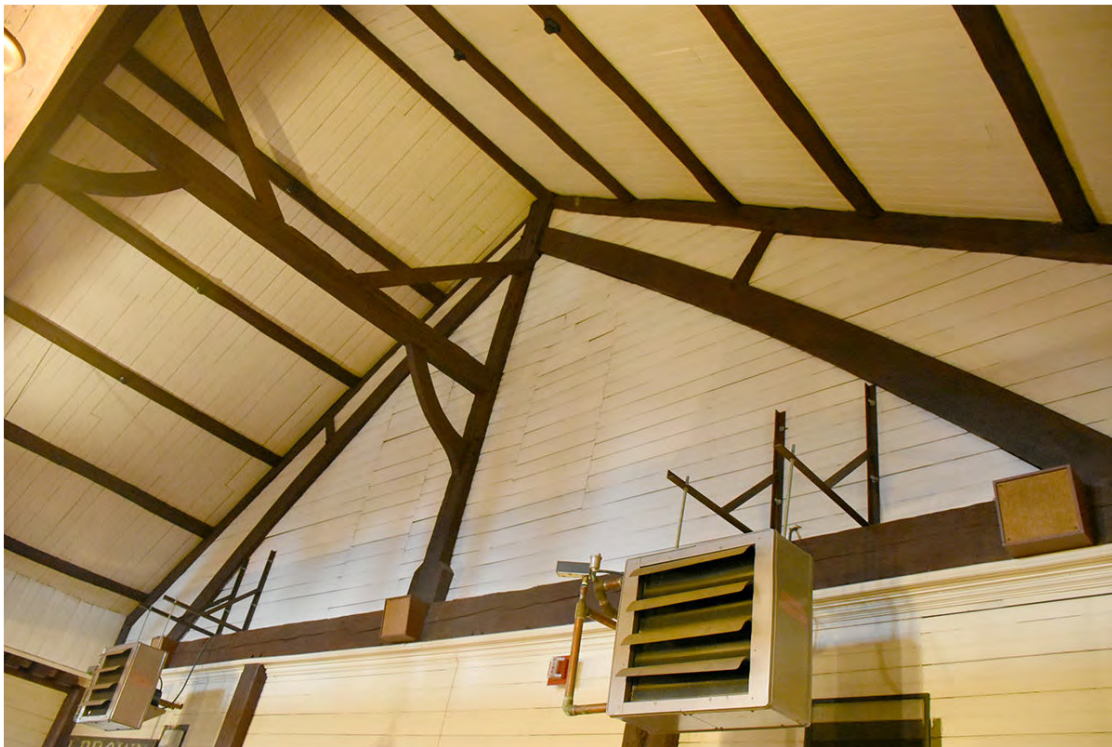
Photo 16: Exposed roof framing in the second-floor hall, north wall. The former openings for the paired arched windows are visible in the beaded matchboard sheathing.
