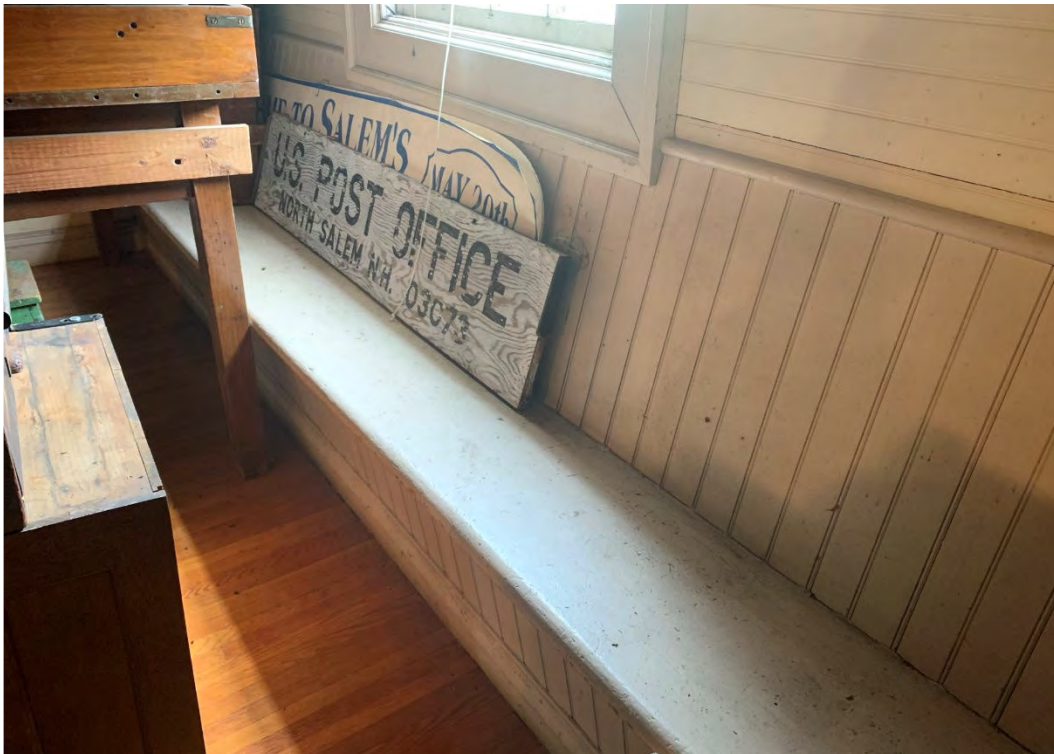
Photo 51: Bench on the west wall of the second-floor hall, showing surface wear through the paint
