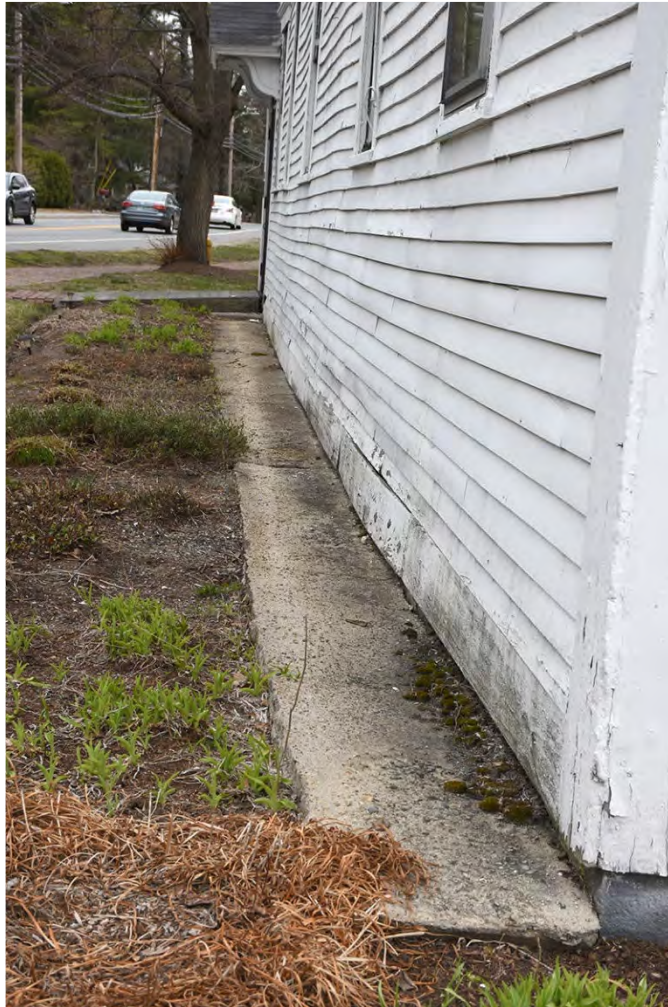
Photo 40: Foundation on the west elevation is mostly hidden by the low water table and the concrete apron installed to protect the foundations from rain runoff from the roof above. Moisture retention is evident in the moss growing along the edge near the foundation.
