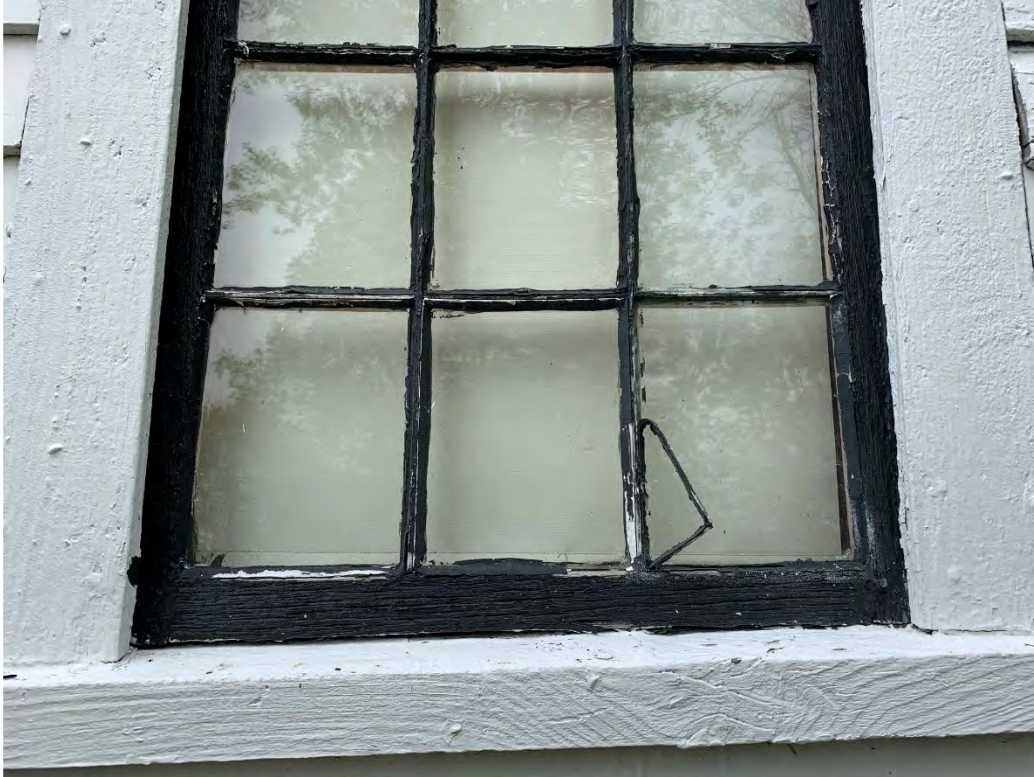
Photo 33: 9/9 double-hung window on the first floor of the east elevation. These may be the oldest surviving windows in the building, potentially dating to the eighteenth century.
