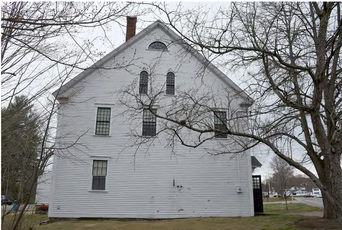
Photo 3: North elevation facing the old Schoolhouse No. 1. This wall was part of the 1908 addition. The windows were reused from the original elevation or added to match existing windows.
