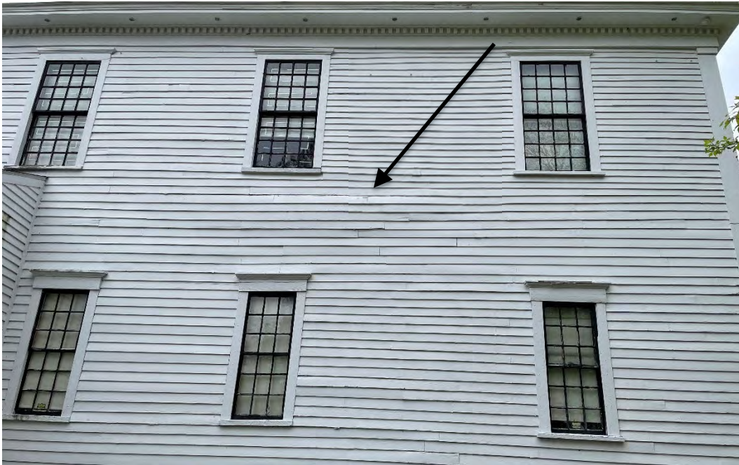
Photo 25: Clapboards in between the first and second floors on east elevation are bulging, indicating a shift in the structure beneath. These clapboards should be removed and repaired or replaced, and the structure checked.
