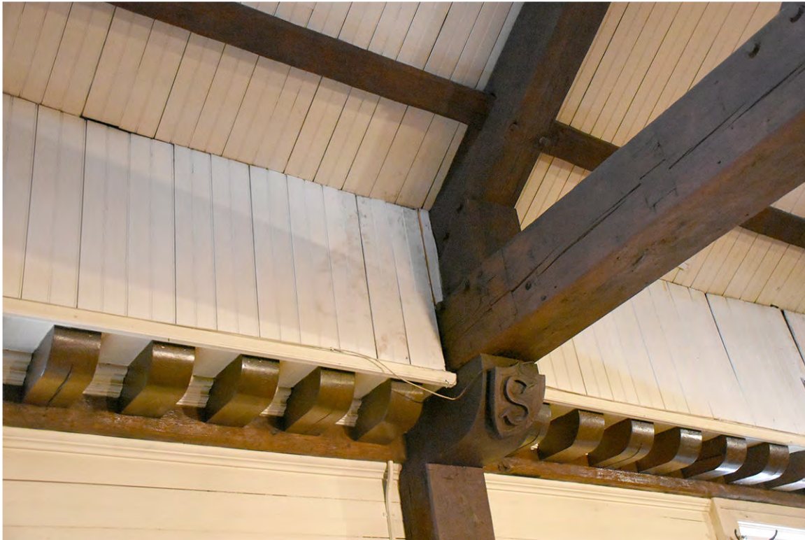
Photo 48: Slight discoloration on the painted beadboard panels adjacent to the carrying beam. Wires and conduit are surface-mounted along trim around the room.
