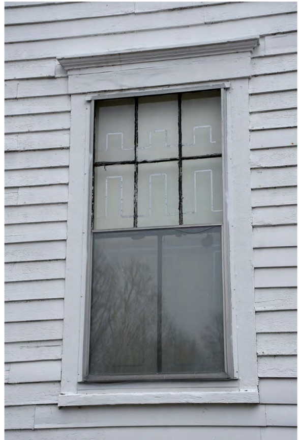
6/2 double-hung windows on the first-floor level.
