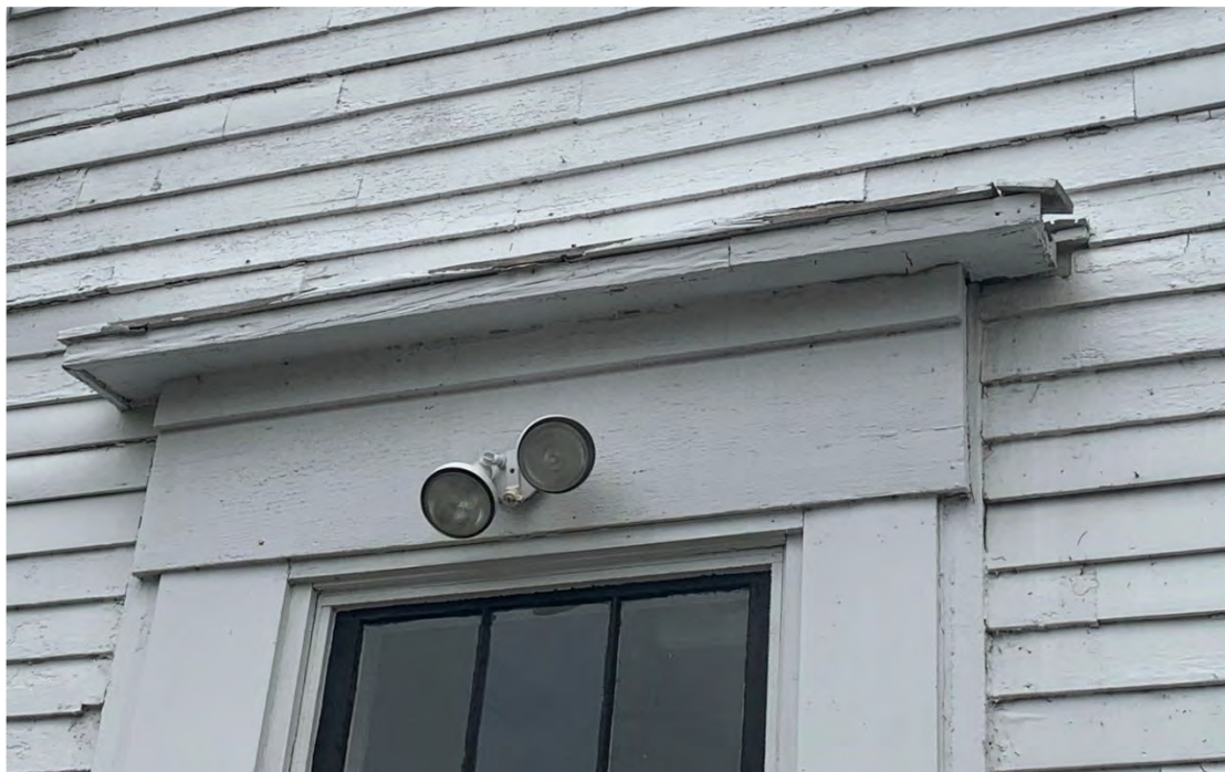
Photo 28: Header and trim molding over the south door are in poor condition.
