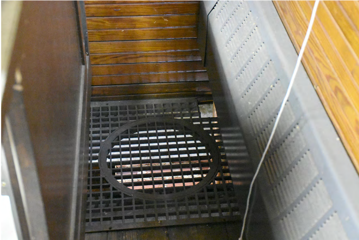
Photo 69: Floor grate for heat and air exchange in the Military Room, north wall, with later radiator panel at right along wall.
