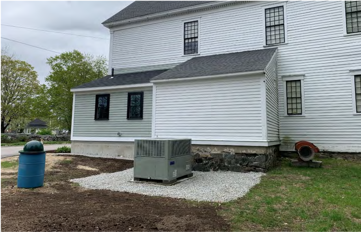
Photo 43: Air conditioning unit newly installed on the east side of the building.
