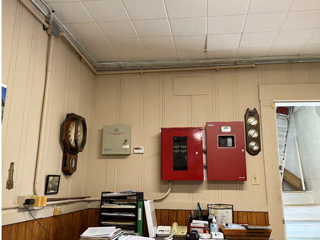
Photo 46: Surface-mounted conduit and wires in the eastern corner of the office.
