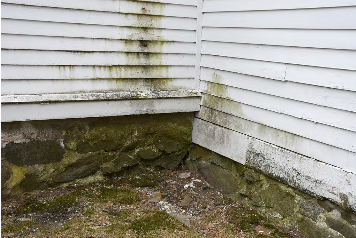
Photo 42: North corner of the shed addition on the east elevation, showing moss and biogrowth on both the foundation and the clapboards, indicating moisture retention.
