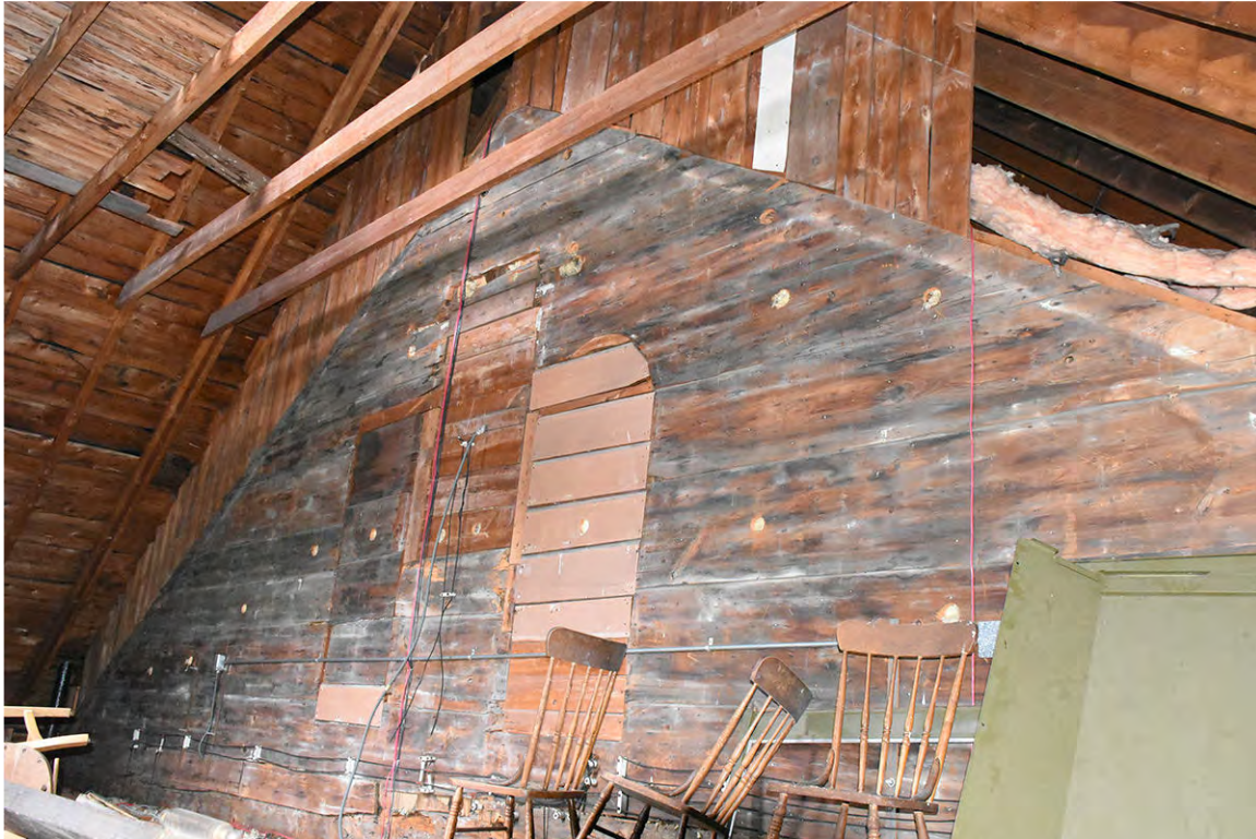
Photo 23: Original north gable end, exterior sheathing exposed in the attic of the north addition. Visible in the sheathing are the original central window, the paired arched windows from 1900, and the ghost lines of the original raking eave boards.
