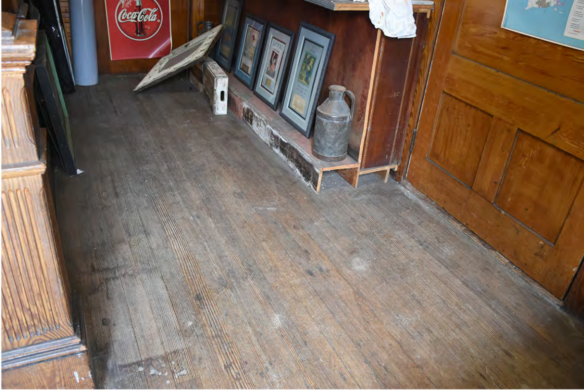
Photo 54: Flooring on the first-floor level of the main entrance on the north end. Surface wear and water staining is visible. The floors need to be refinished with a protective clear coat of varnish.
