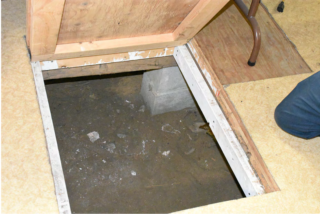
Photo 45: Trap door in floor of the main room providing access to the crawlspace. Area is clean and dry, and CMU blocks supporting floor structure are visible.
