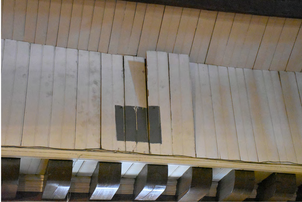
Photo 50: Beadboard panels in the southeast corner show displacement, painted ghost of the former location of a PA speaker.
