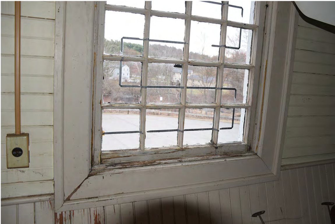
Photo 59: Window interior in the east wall of the second-floor main room. Interior sills were removed in the 1900 renovation. Deterioration and water damage is apparent in the lower sash and trim.
