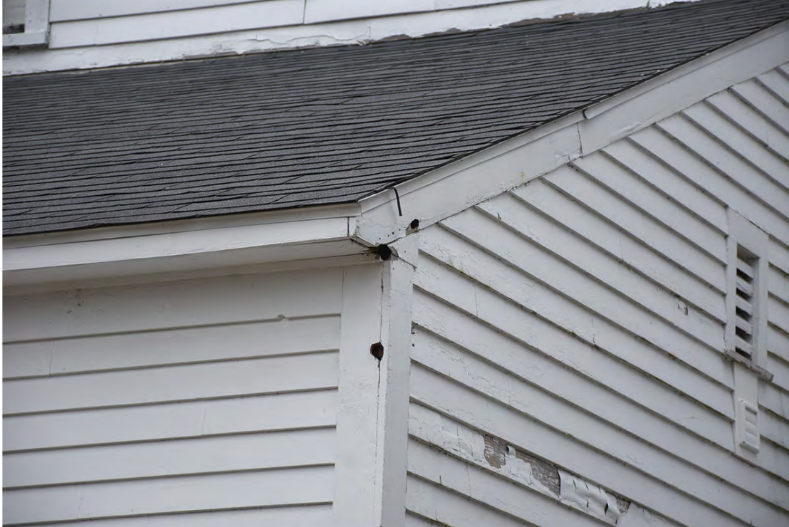
Photo 27: Insect or animal holes in the trim on the northeast corner of the vault addition. Peeling paint is seen on the clapboards facing north.
