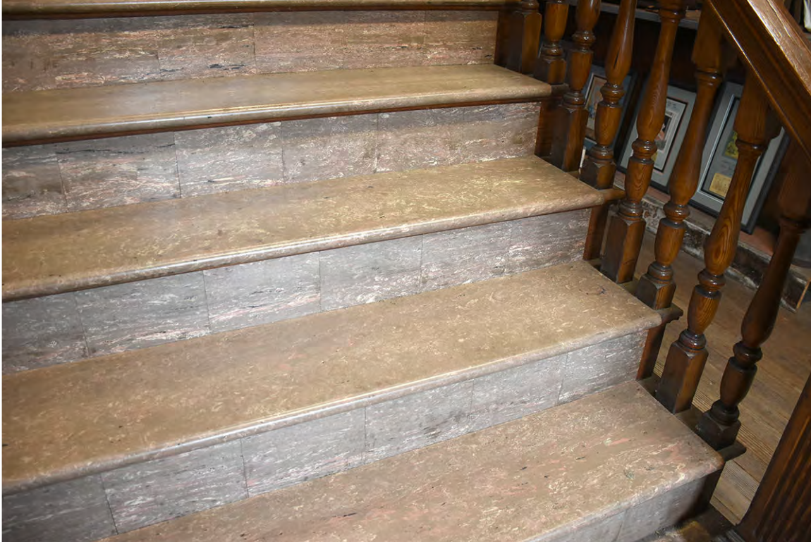
Photo 53: Linoleum covering the treads and risers of the main staircase.
