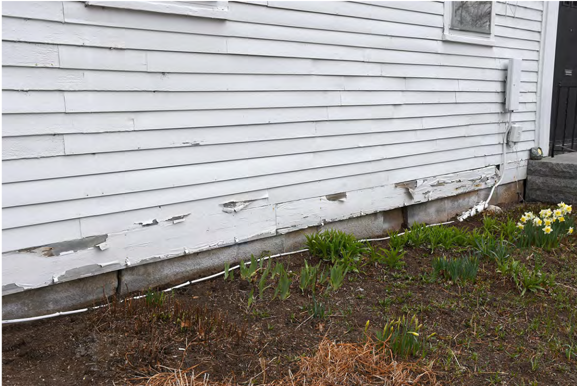
Photo 41: Granite foundation blocks on the south elevation are displaced and have missing mortar. They also have a fine layer of white paint sprayed on the surface, likely spillover from a previous painting campaign. Plantings should be pulled back from the foundation walls.
