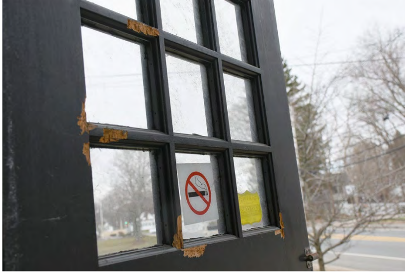
Photo 36: Interior of the main entry doors, recent damage possibly by rodents.
