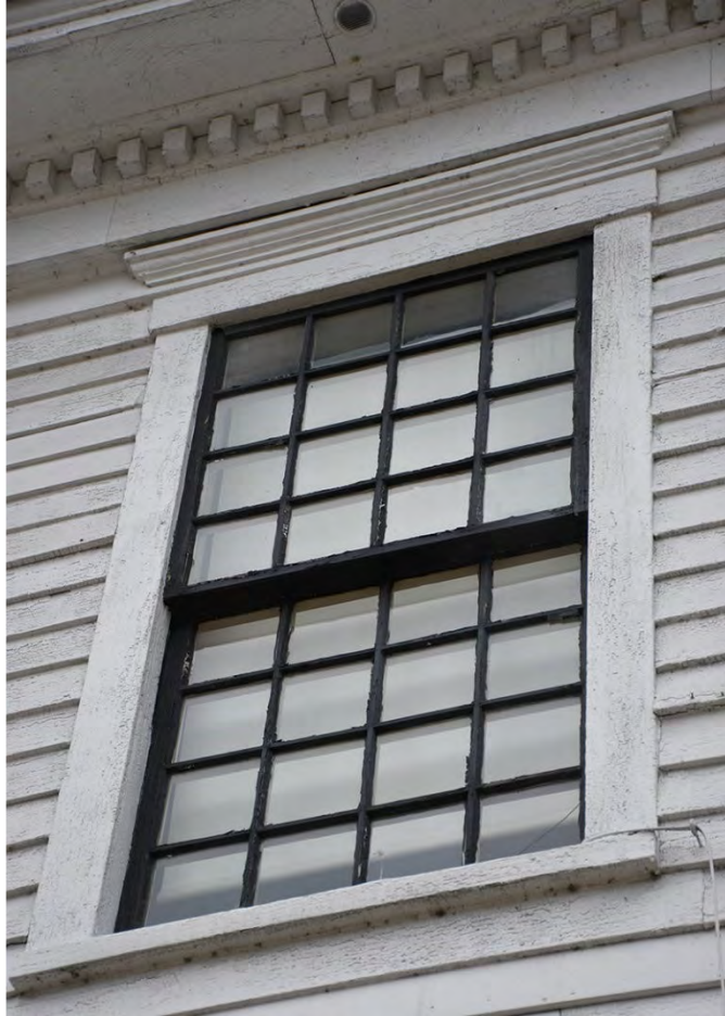
Photo 32: 16/16 double-hung window at the second-floor level of the west elevation. Glazing putty is in poor condition, and lower right pane of glass is cracked. Early twentieth century trim cap was added to the fascia board above the header.
