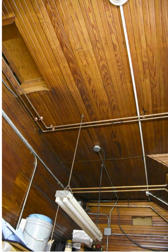
Photo 55: Ceiling of the kitchen, looking west, with conduit and pipes mounted on the surface of the wood beadboard panels.
