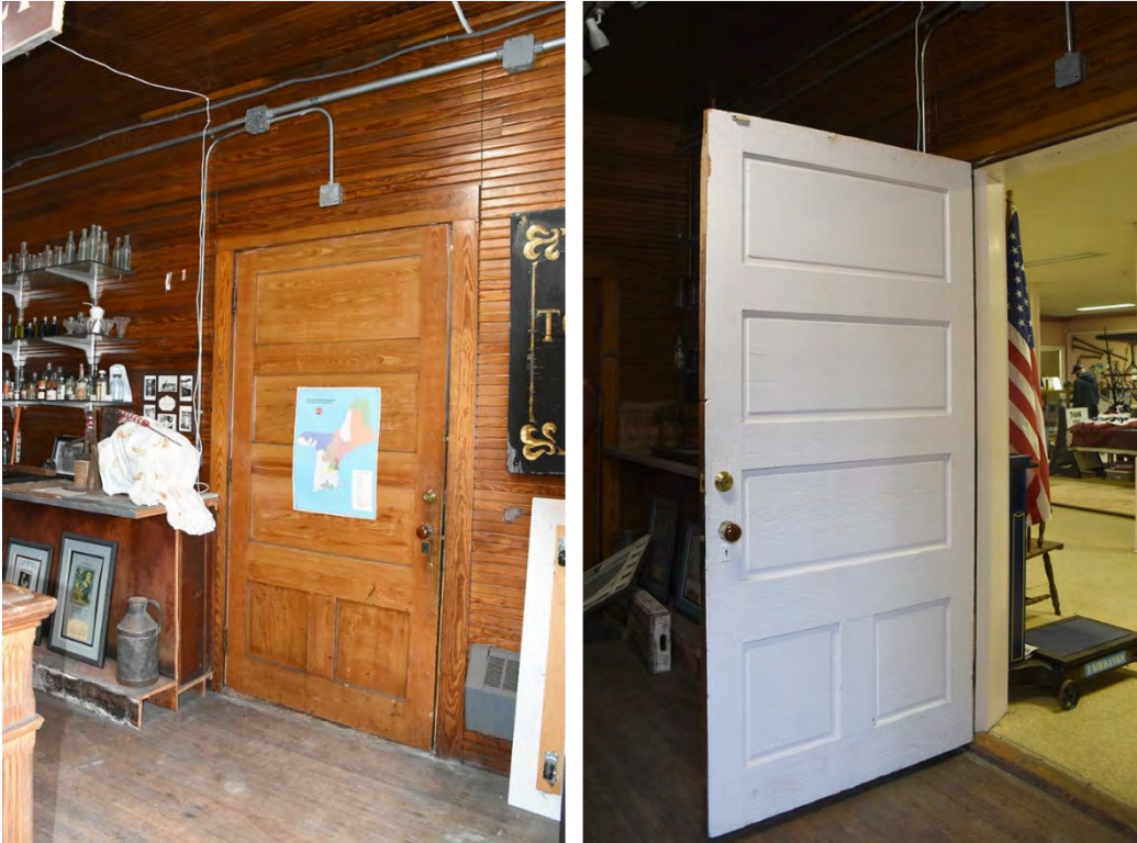
Photo 63: Five-panel door from the main entrance into the first-floor town hall room. Wear and surface abrasion is apparent on the corner and around the doorknob and lock.
