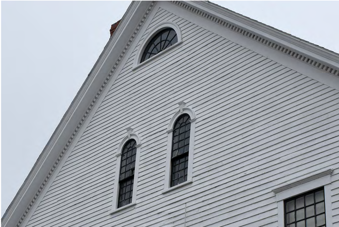
Photo 34: South elevation, paired arched windows and lunette within the gable are twentieth century additions. Glazing putty on each window is visibly lifting or missing.
