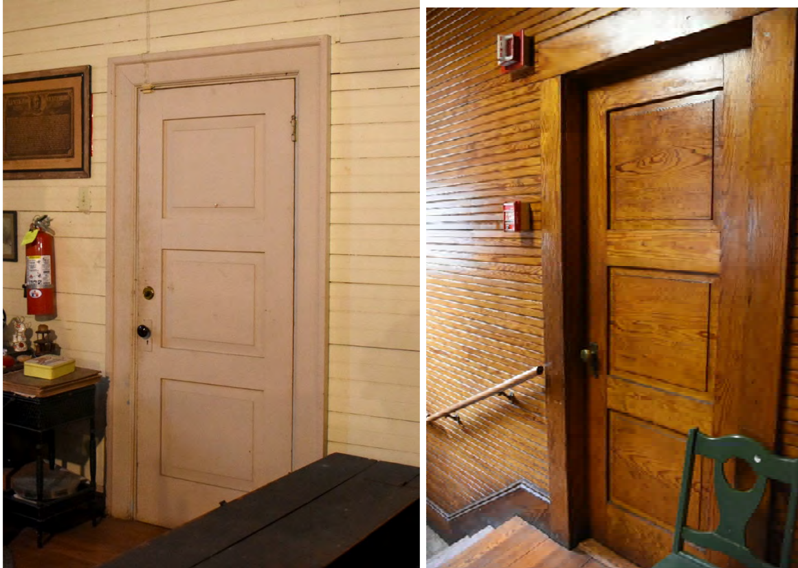
Three-panel doors on the second floor.
