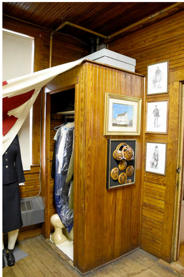
Photo 21: Water closet in the "Military Room", now used as a storage closet. Vent pipe still remains, extending through the roof.
