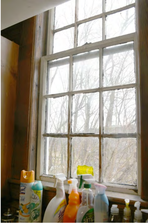
Window interior of 9/9 window on east wall in kitchen Photo 61: (left) and in the main room Photo 62: (right). Muntins have severe deterioration, and upper and lower sash do not meet properly. Window muntins differ, showing the use of sash from different time periods.
