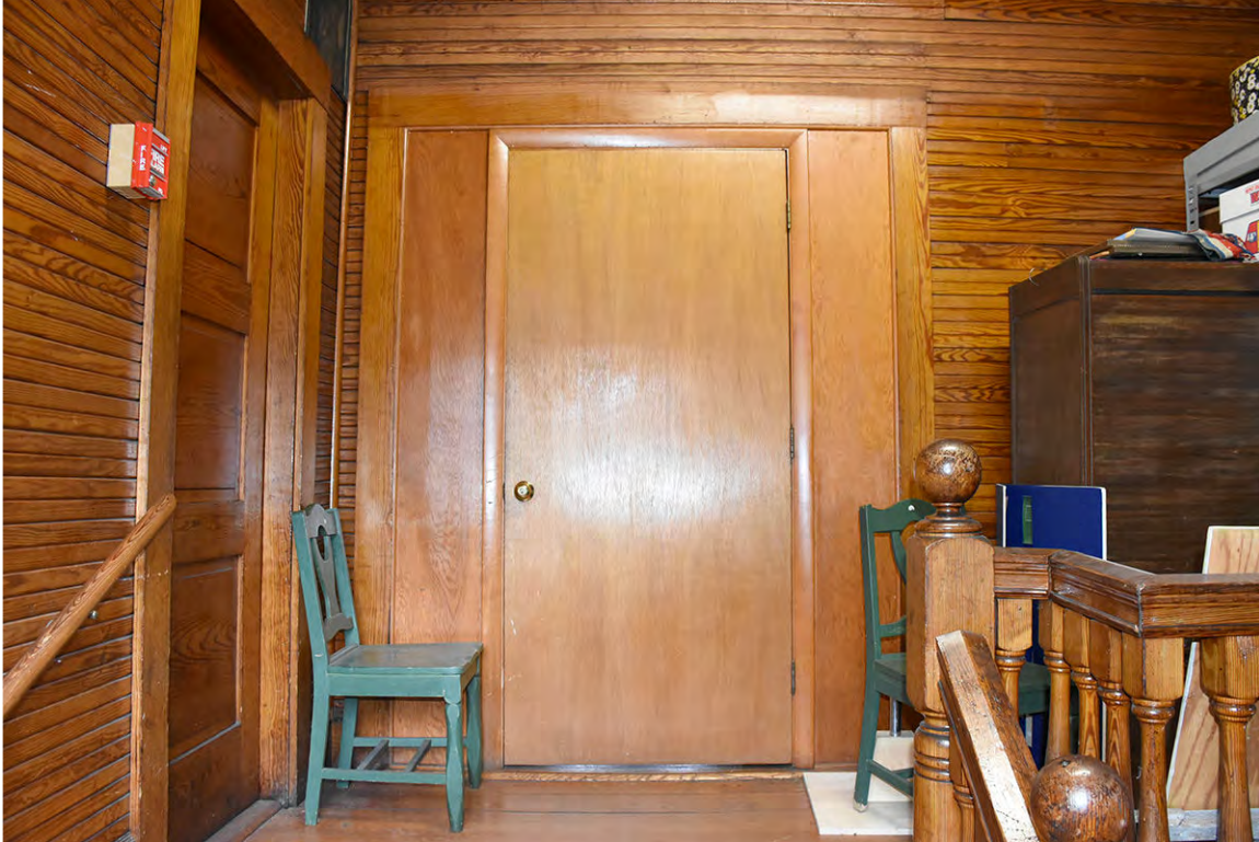
Photo 66: Main doorway into the second-floor hall was infilled in the mid-twentieth century with a flat hollow-core door. A 1908 3-panel door into the Military Room space is at left.
