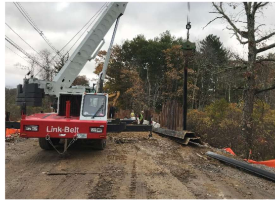
Removing Temporary Cofferdams
