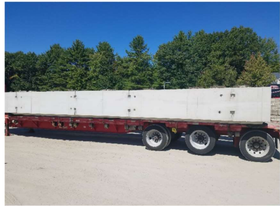
Completed Bridge Segment at Michie Corp Precast Plant Ready to be Trucked to the Site
