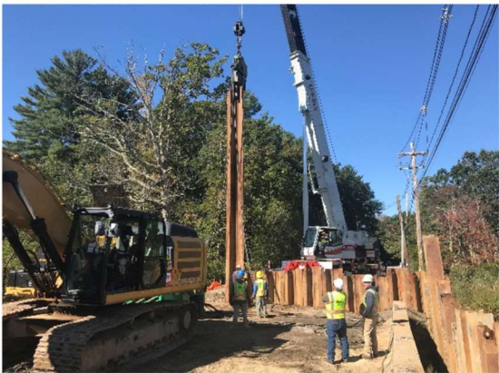
Building the "Wall" Which will be Removed Once the Bridge is Build
