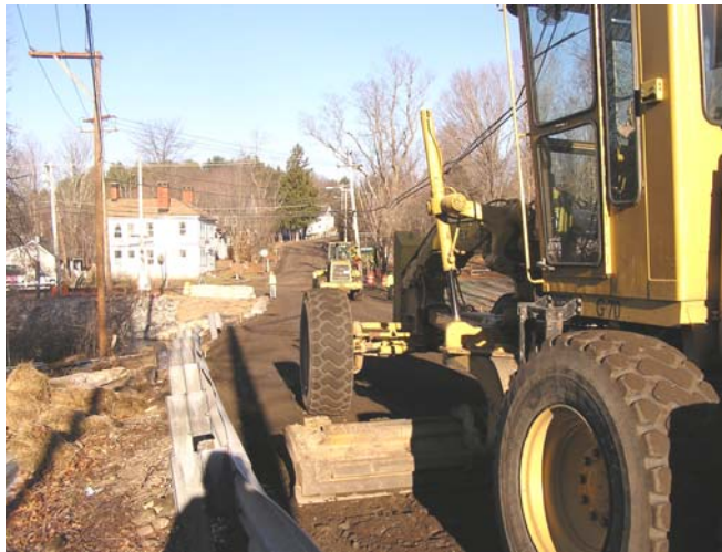
grading and compacting road gravels
