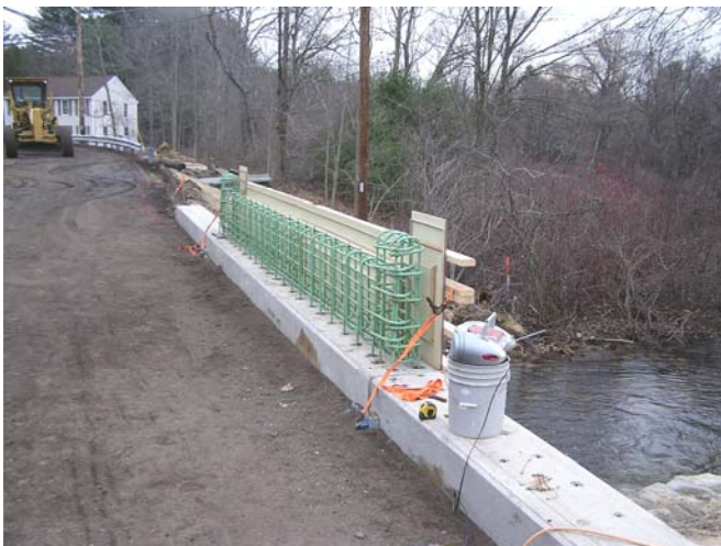
bridge rail reinforcing steel
