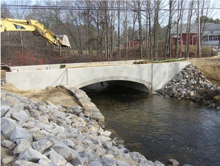
At Left Looking Upstream at New Bridge: Restoration of natural stream flow; diversion pipe removed and stone protection in place.
