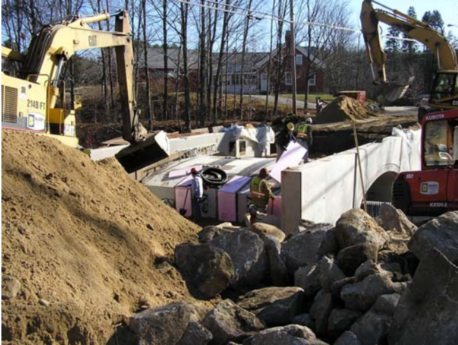
Backfilling against new precast bridge
