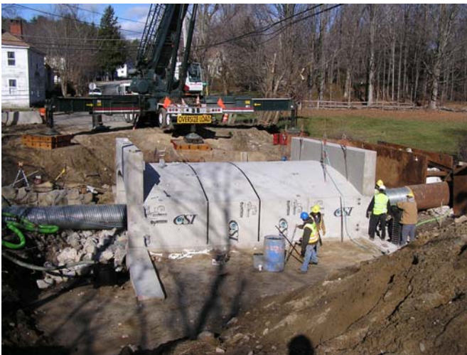
Installation of Precast Concrete Bridge Sections (above)
