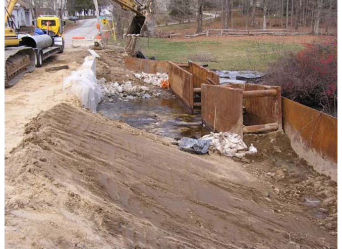
Side slope prep prior to stone placement
