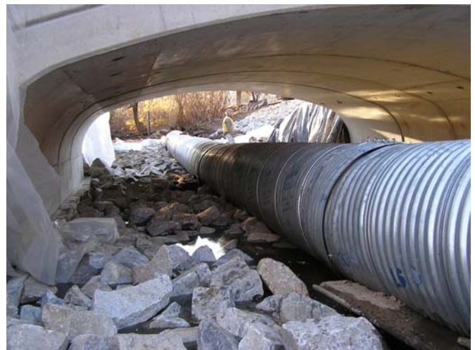
View underneath new bridge structure with stream bypass pipe still in place (above)
