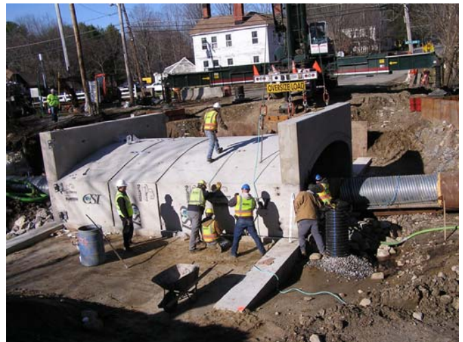
Installation of Precast Concrete Bridge Sections (above)
