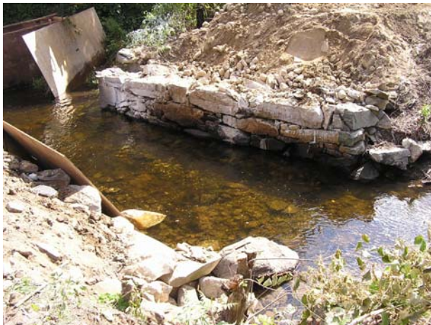
Old Stone Bridge Abutment Prior to Removal
