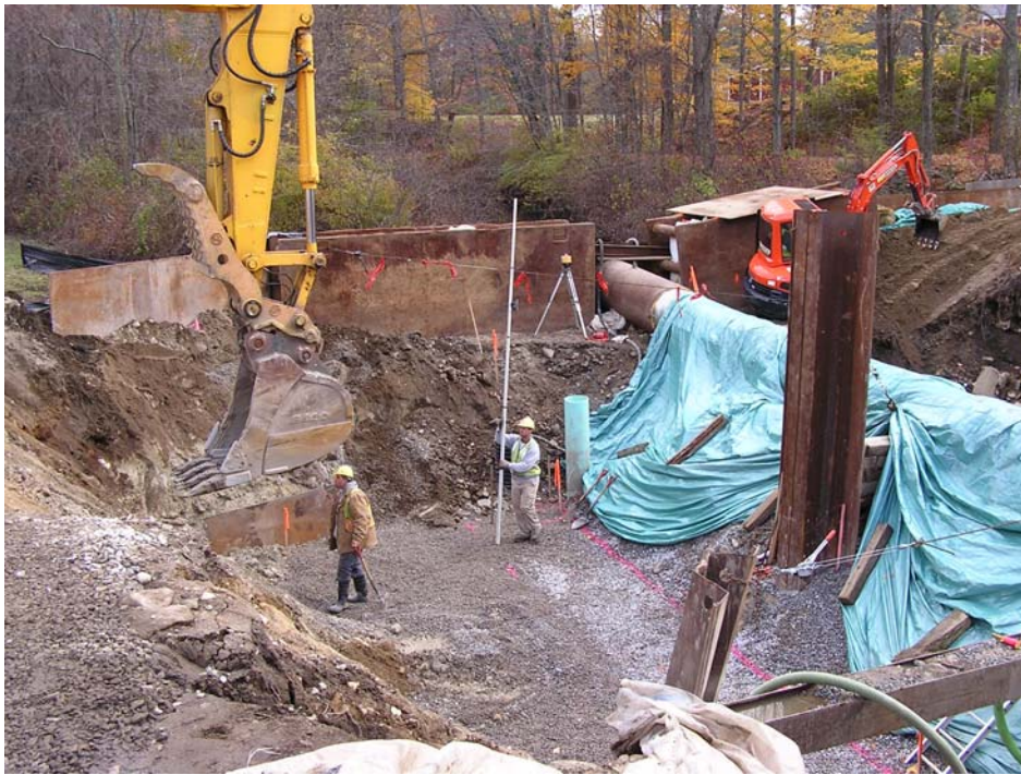
Excavated Area Being Prepared for New Footing
