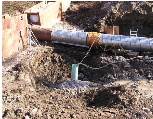
Stream Bypass Piping and Dewatering Pit
