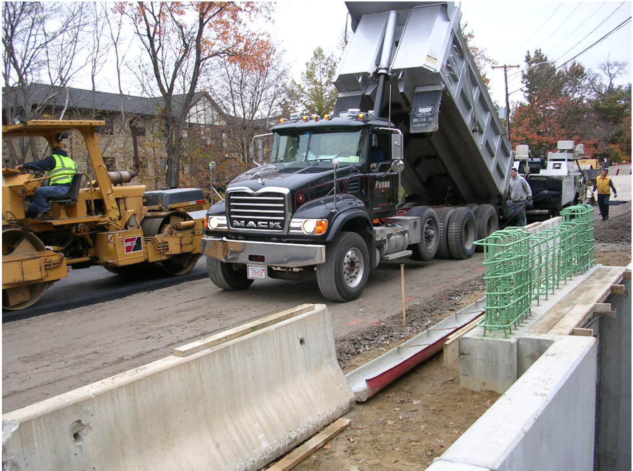
Base Course Paving Operation
