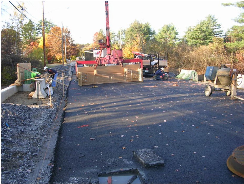
Setting Bridge Rail Formwork
