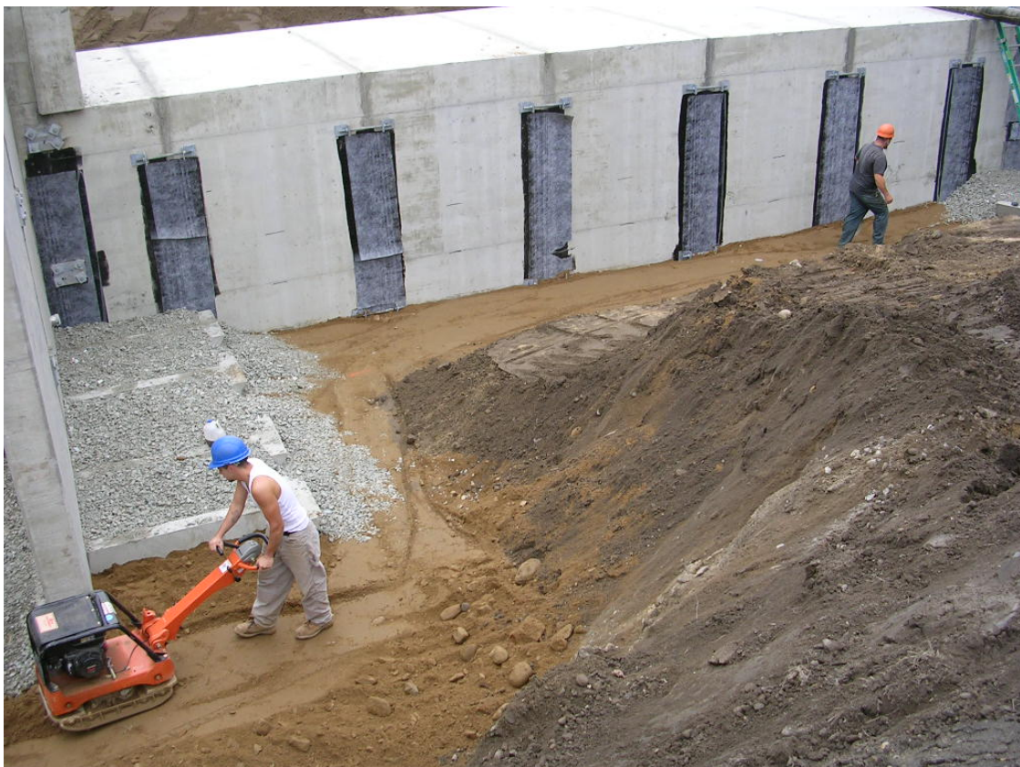
Backfilling box and wing walls
