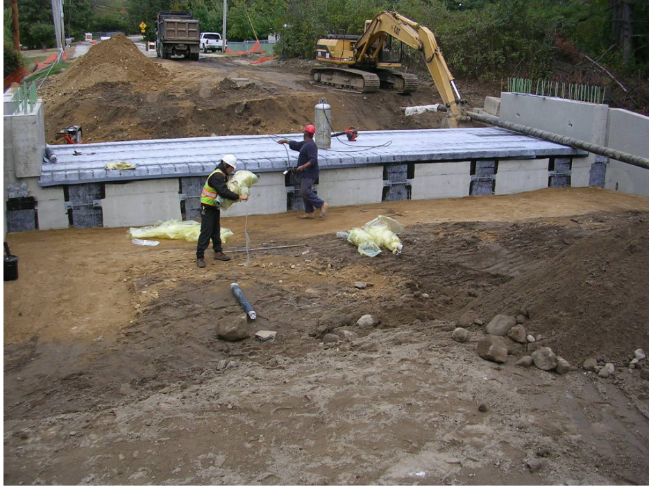
Installing barrier membrane
