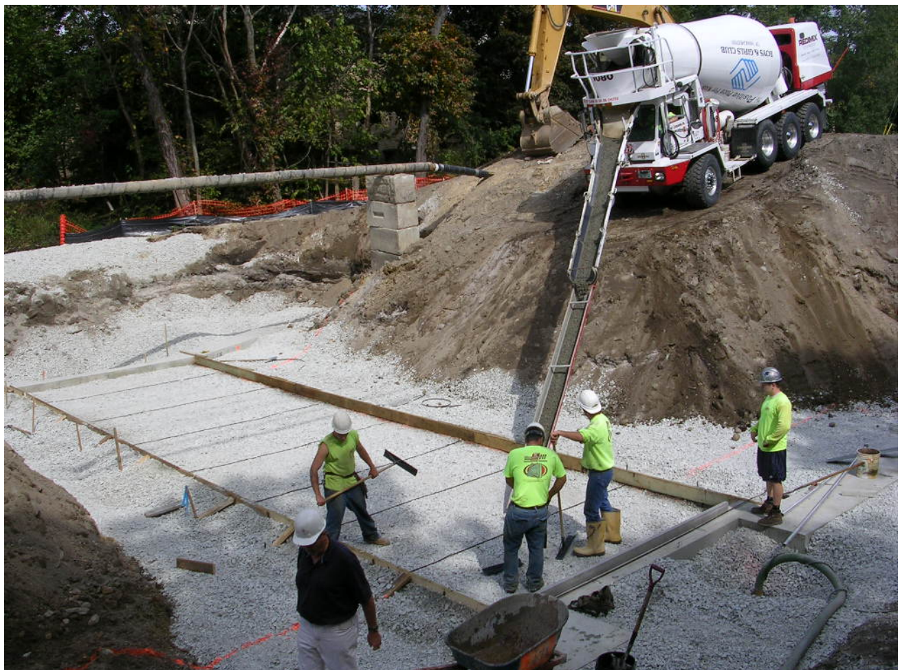
Pouring concrete mudslab
