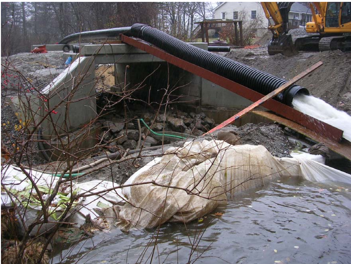
Large dewatering pump installed to pass streamflows.
