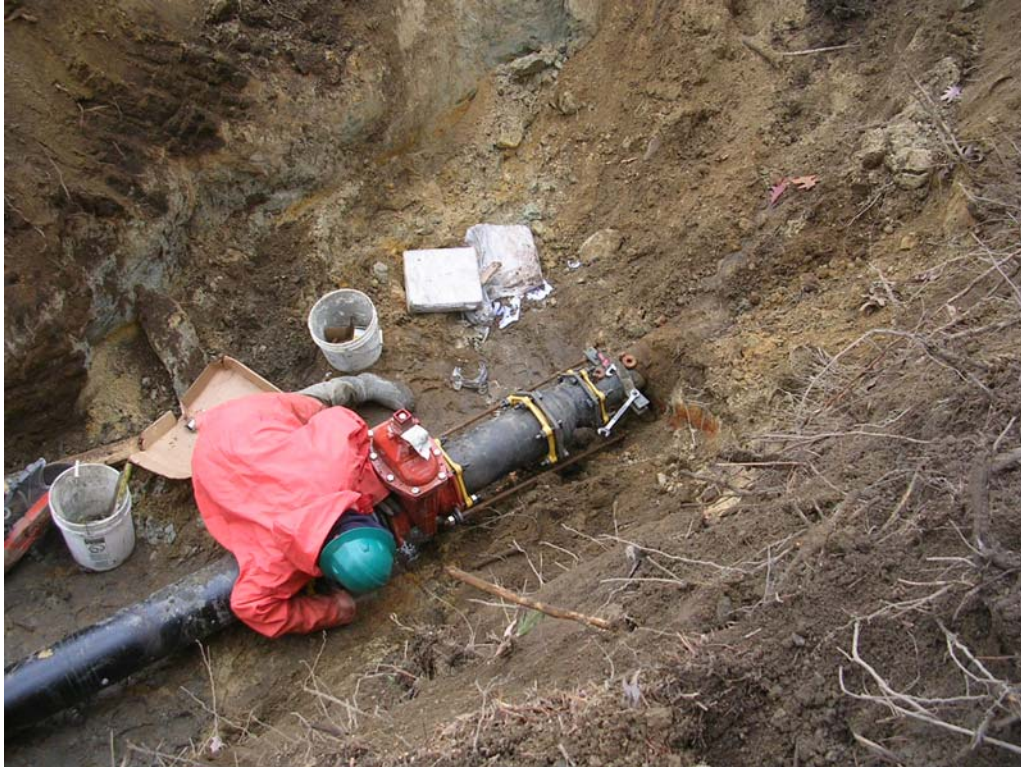
Contractor installed reducer and gate valve in order to restore water to residents.
