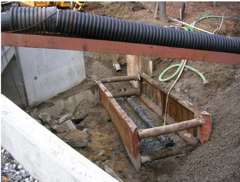
Contractor uses trench box to maintain excavation during waterline installation.
