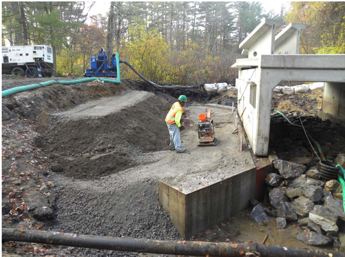
Contractor placing structural backfill along bridge sides and footings.
