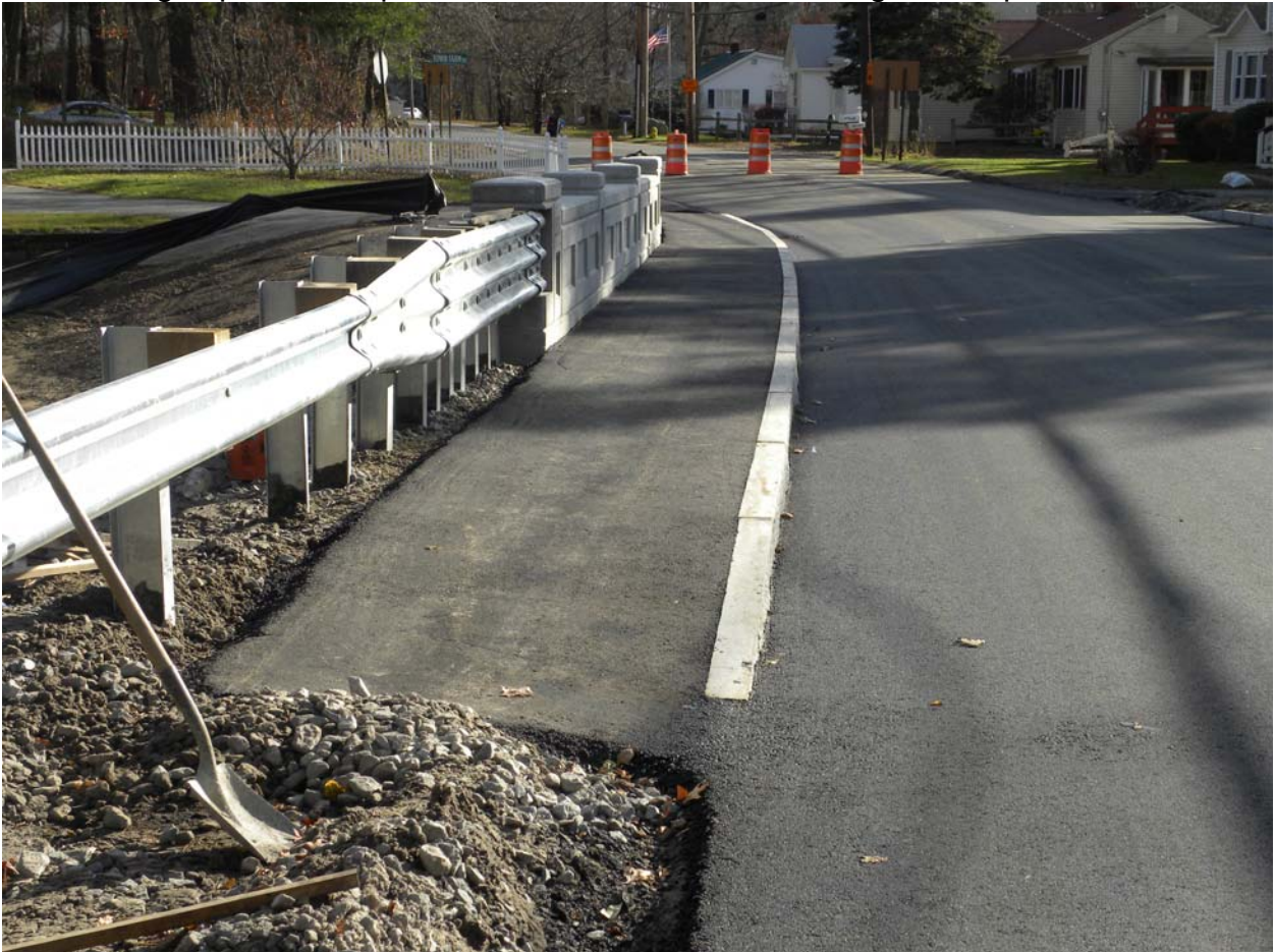
Final pavement on roadway and sidewalk.
