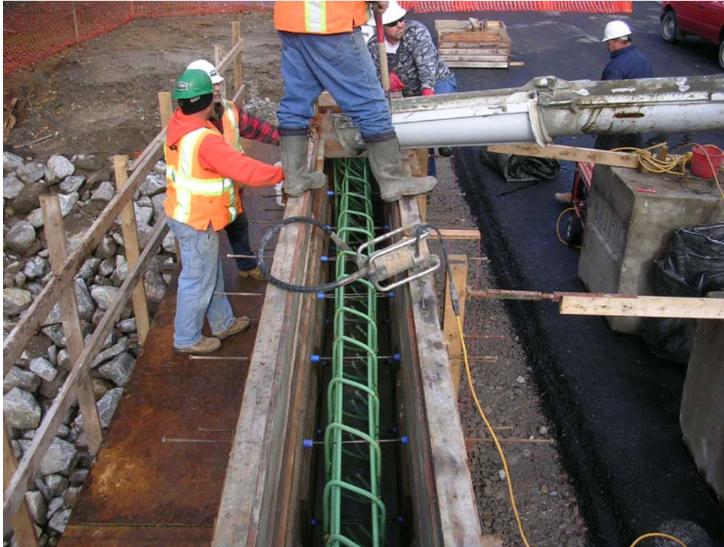
Contractor placing final concrete railing section.
