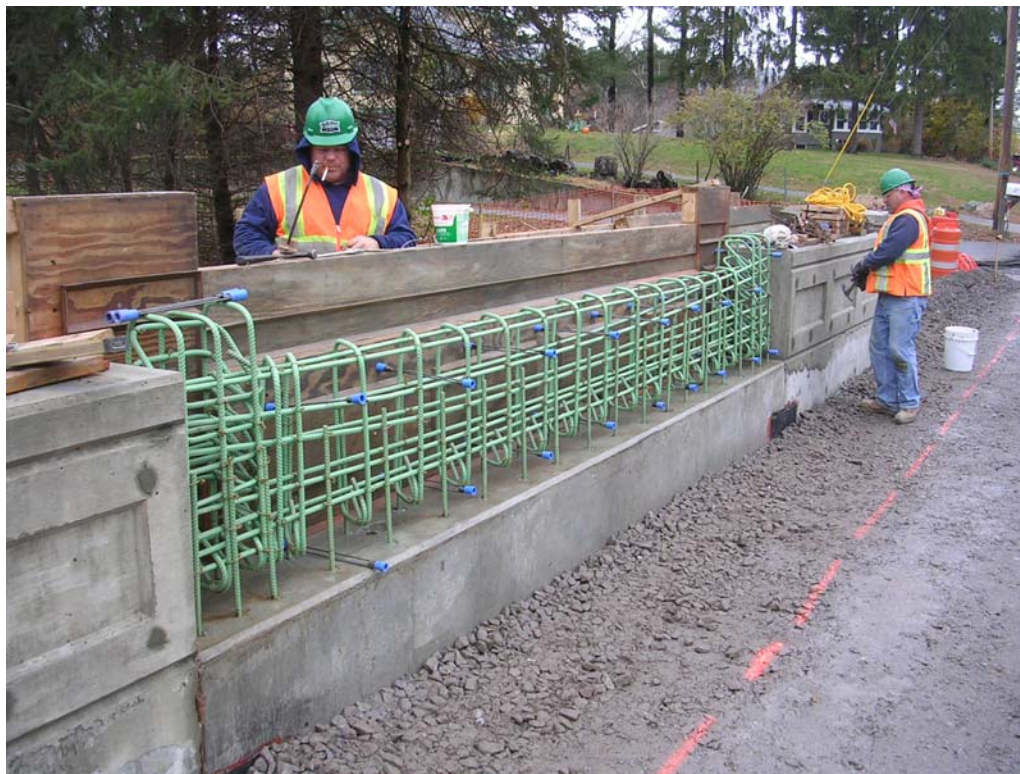
Contractor installing rebar and decorative formwork for cast-in-place concrete railing.
