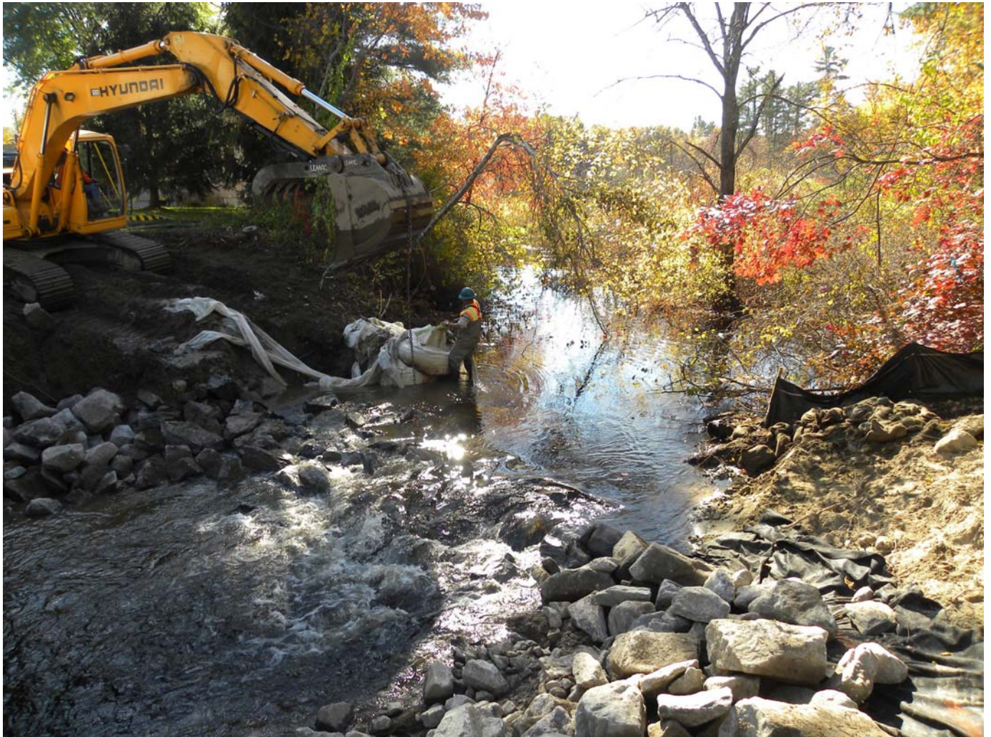
Contractor removing cofferdam to allow natural streamflow again.
