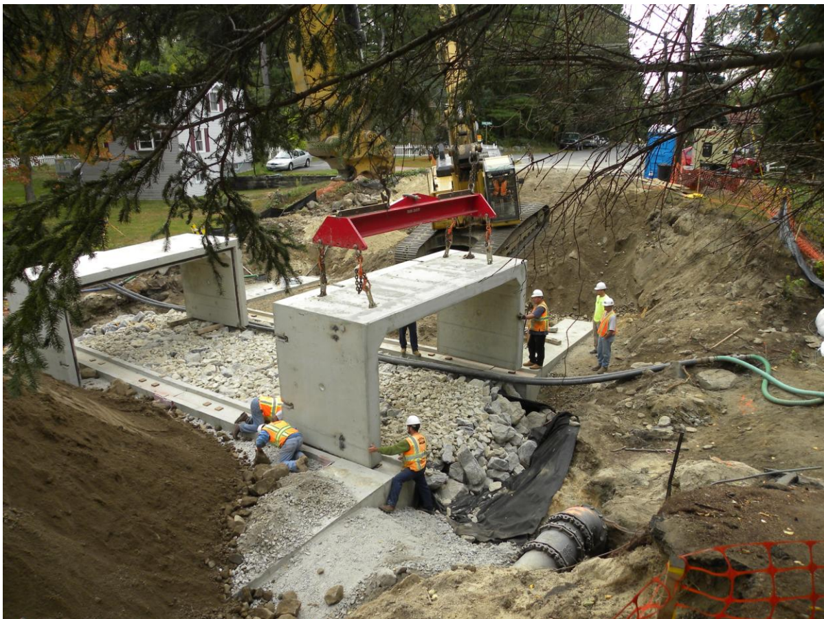
Contractor positioning the first piece of the pre-cast rigid frame.
