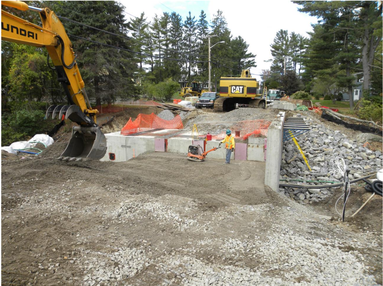
Pre-cast elements majority complete. Downstream embankments taking shape.
