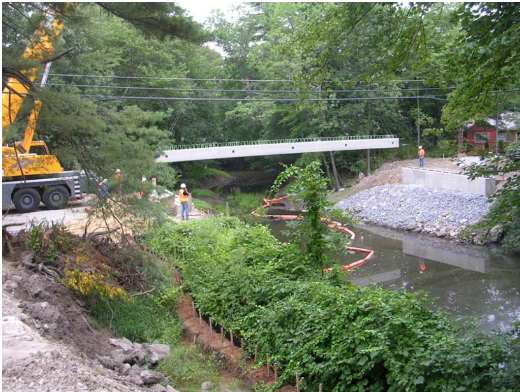
Setting first concrete box beam
