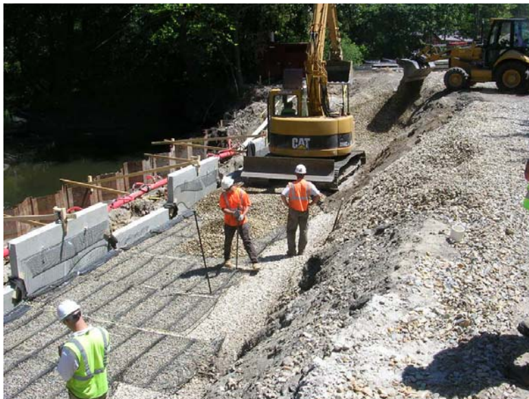
Installing MSE retaining wall
