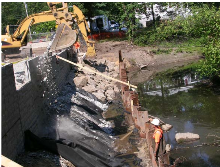
Placing rip rap in front of MSE retaining wall
