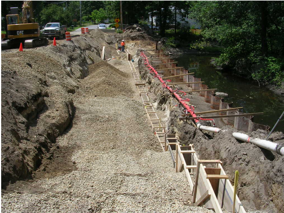
Forming the MSE wall leveling pad
