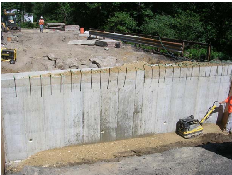
Backfilling east abutment
