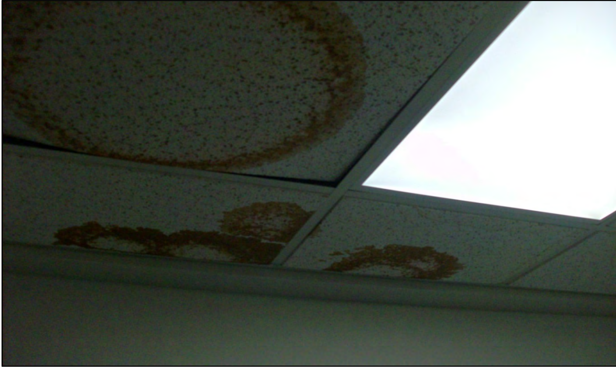
Stained ceiling tiles in bathroom from roof leaks.
