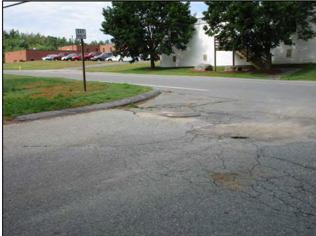
Exit driveway at intersection with Geremonty Drive. Cracking, differential settlement. Note undersized sign.
