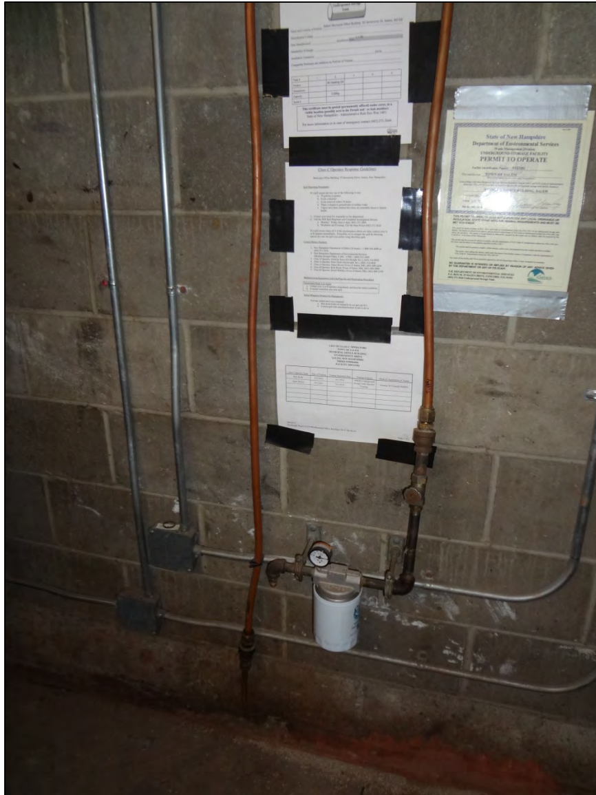
Abandoned oil piping and signs to remove.
