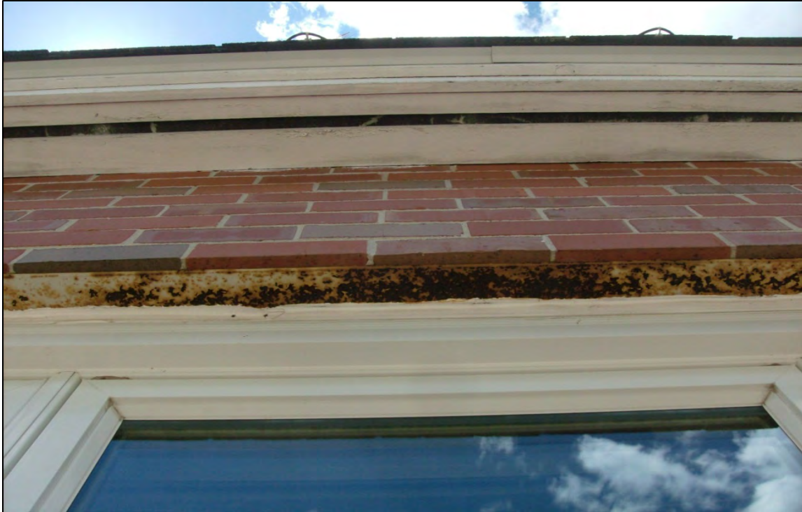
Typical condition of rust on lintels over windows.
