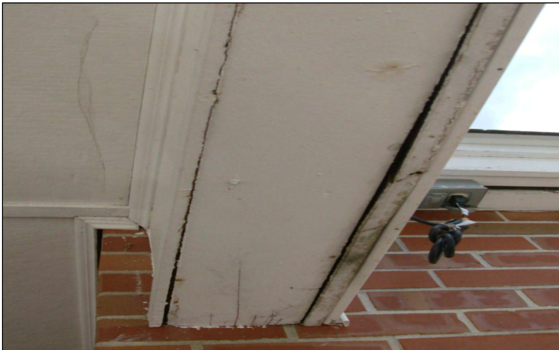
East side beam enclosure is separating at canopy and there is some rot starting.
