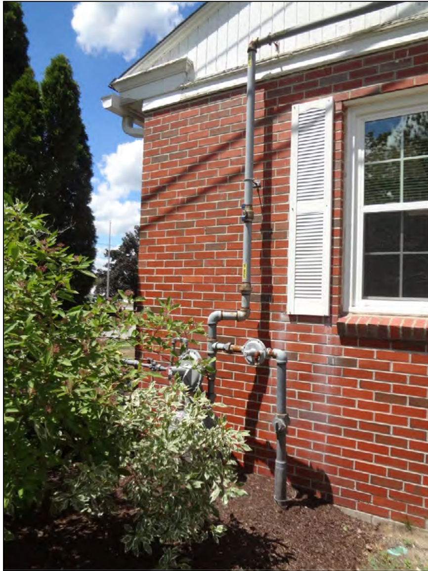
Gas regulator close to window.
