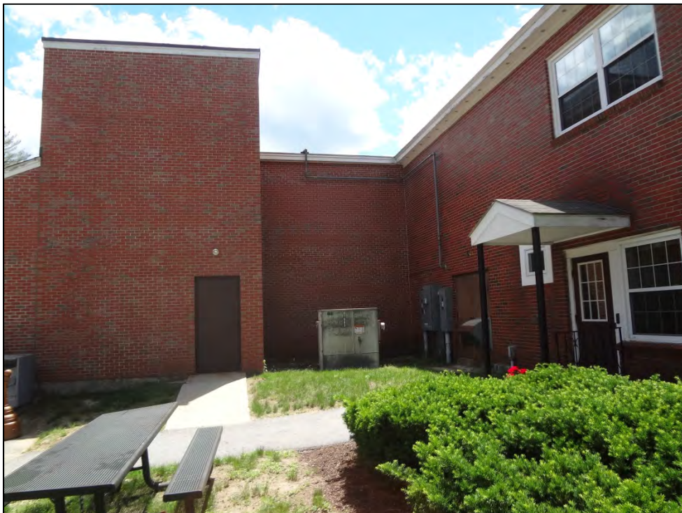
Gas line on side of building prone to ice damage. Ladder location potential.
