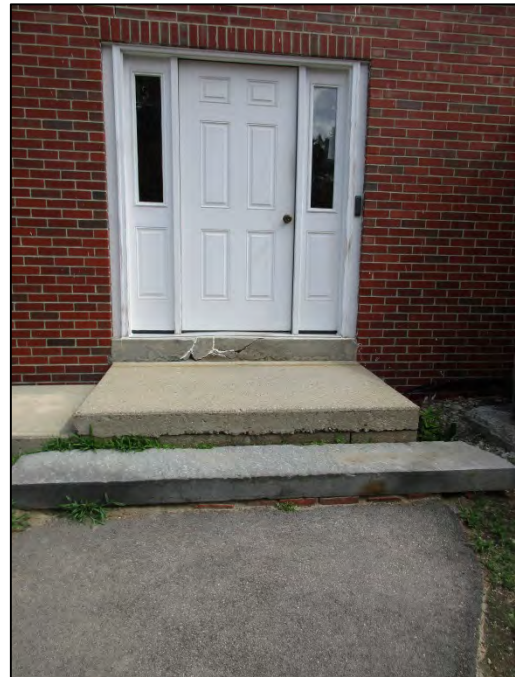
Stairs at southwest entrance. Replacement required for compliance with ADA. Note absence of handrails.
