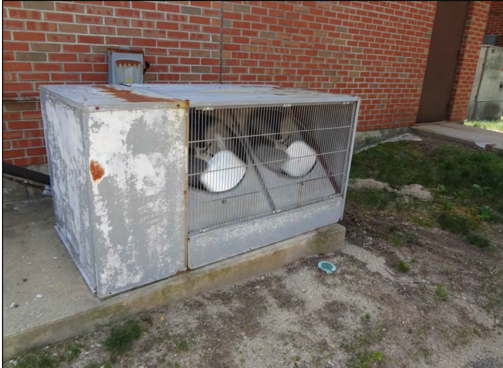
Older cooling unit in need of replacement.
