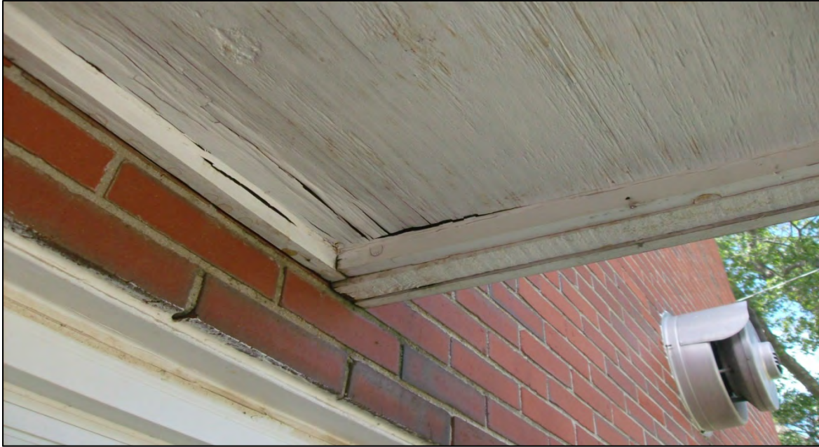
Rotted ceiling board under canopy at finance department entry door.
