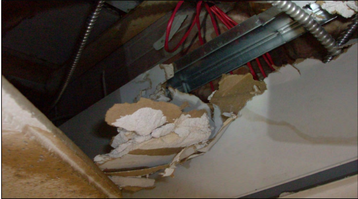
Damage to gypsum above suspended ceiling in community development area from water damage.
