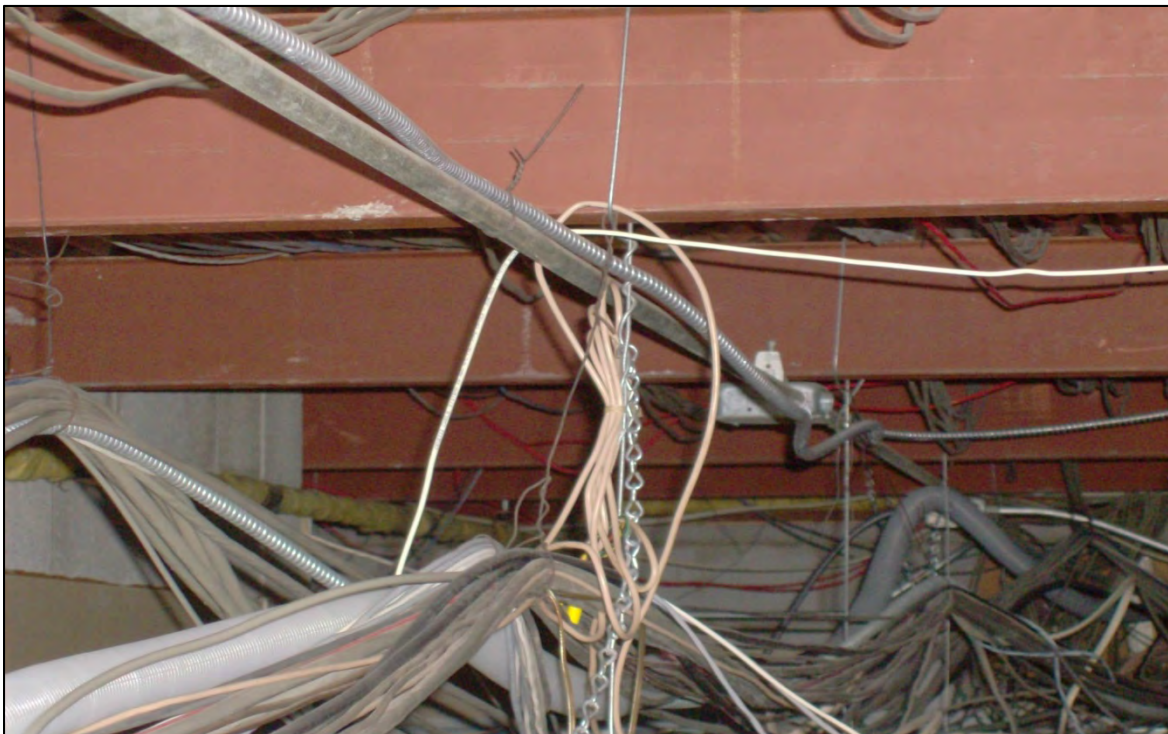
Tangle of wiring and communication cables over corridor ceiling. Many cables are no longer used.
