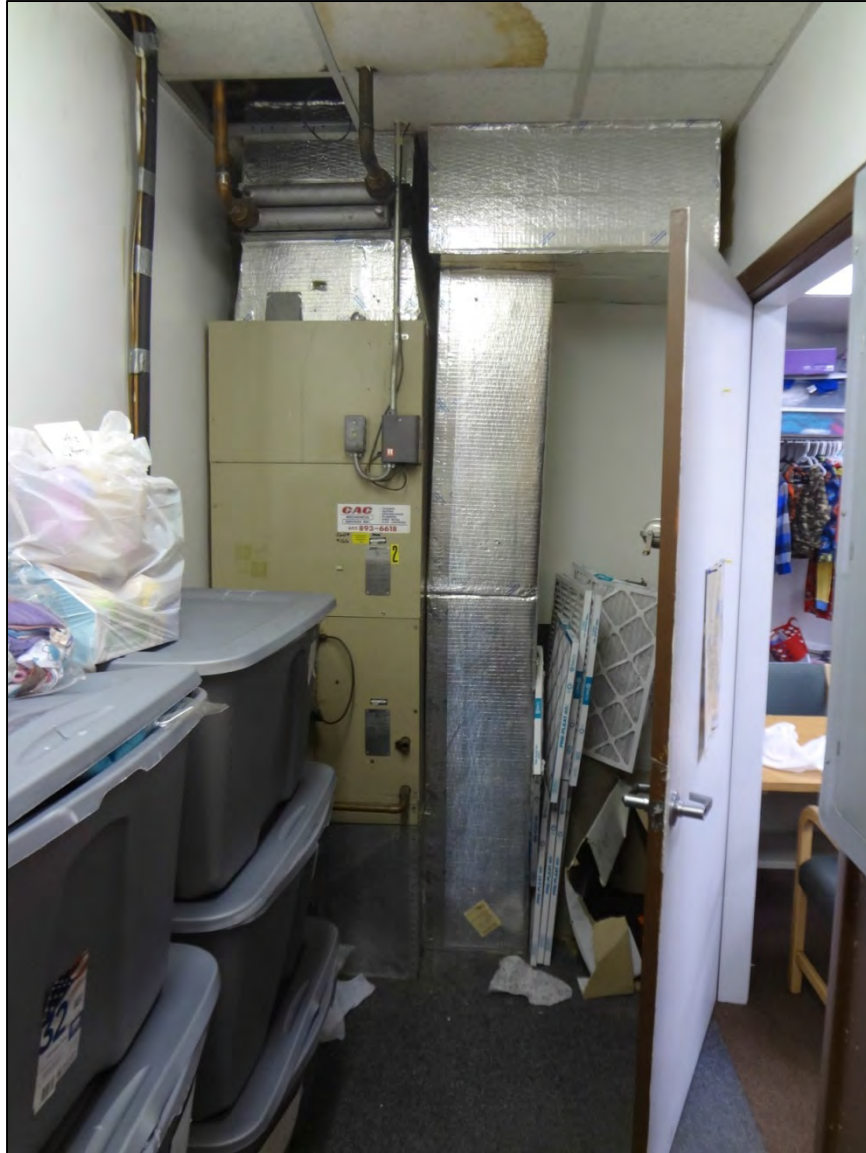
Typical air handling unit in a closet space.
