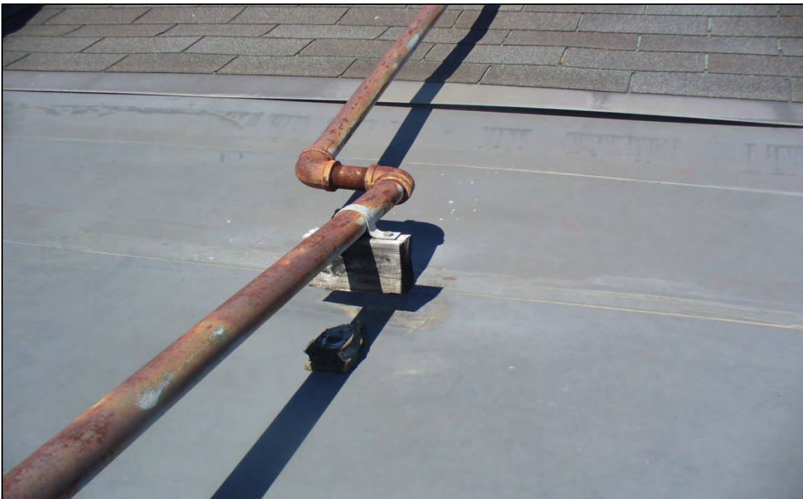
Gas line runs from attic space to mechanical units on roof and over to boiler room.
