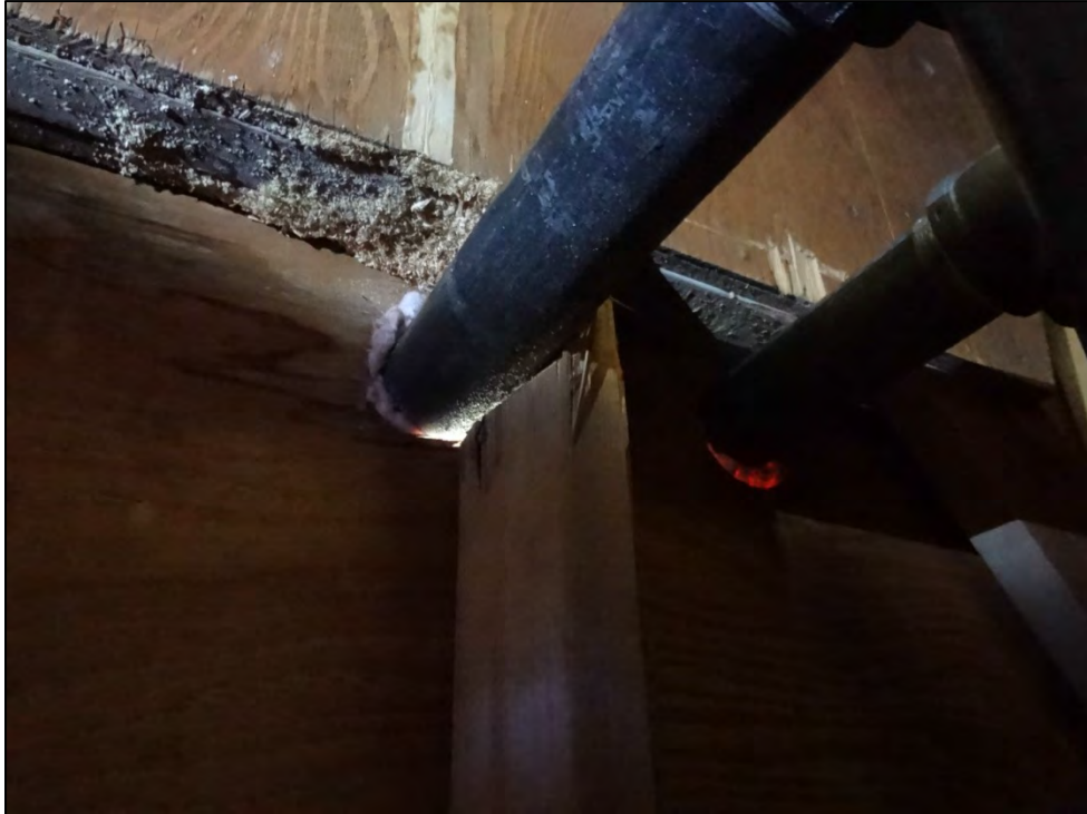
Gas line penetration through gable end.
