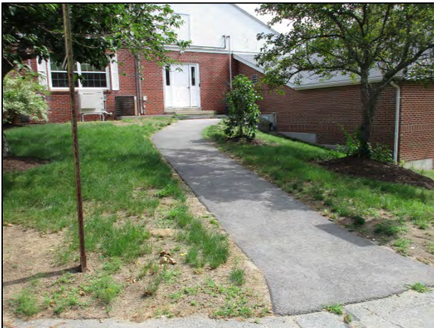
Sidewalk with 10% slope; no railings or landings.
