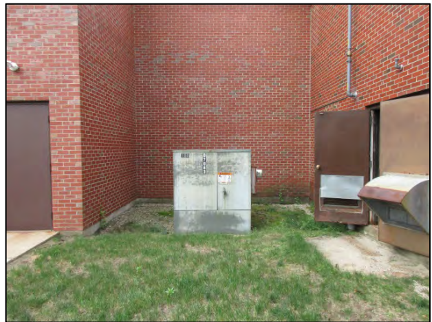
Transformer location. No means to drain away runoff.
