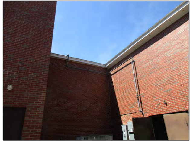
Gas line on north side prone to ice encapsulation.
