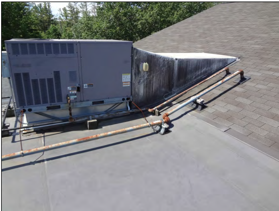
Gas piping needs repainting and supports.
