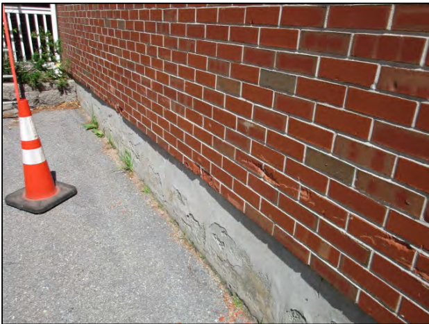
Damage to the brickwork from vehicle impacts. Bollards or a guardrail can protect the building from future damage.
