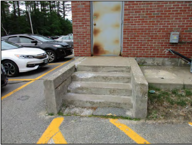
Deteriorating concrete at northeast stairs and landing. Also note absence of guardrails and handrails.
