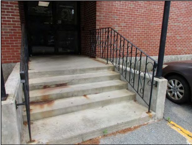
Non-ADA railings. Note cracked concrete riser and staining from corroding reinforcement steel.
