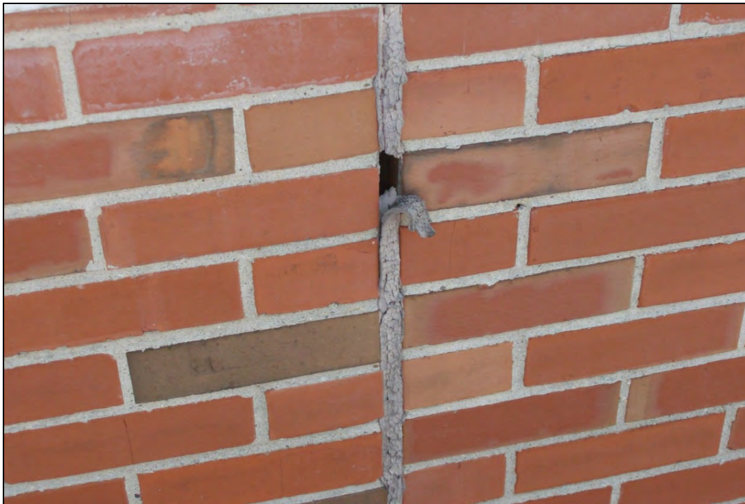
Deteriorated and failed control joint sealant.
