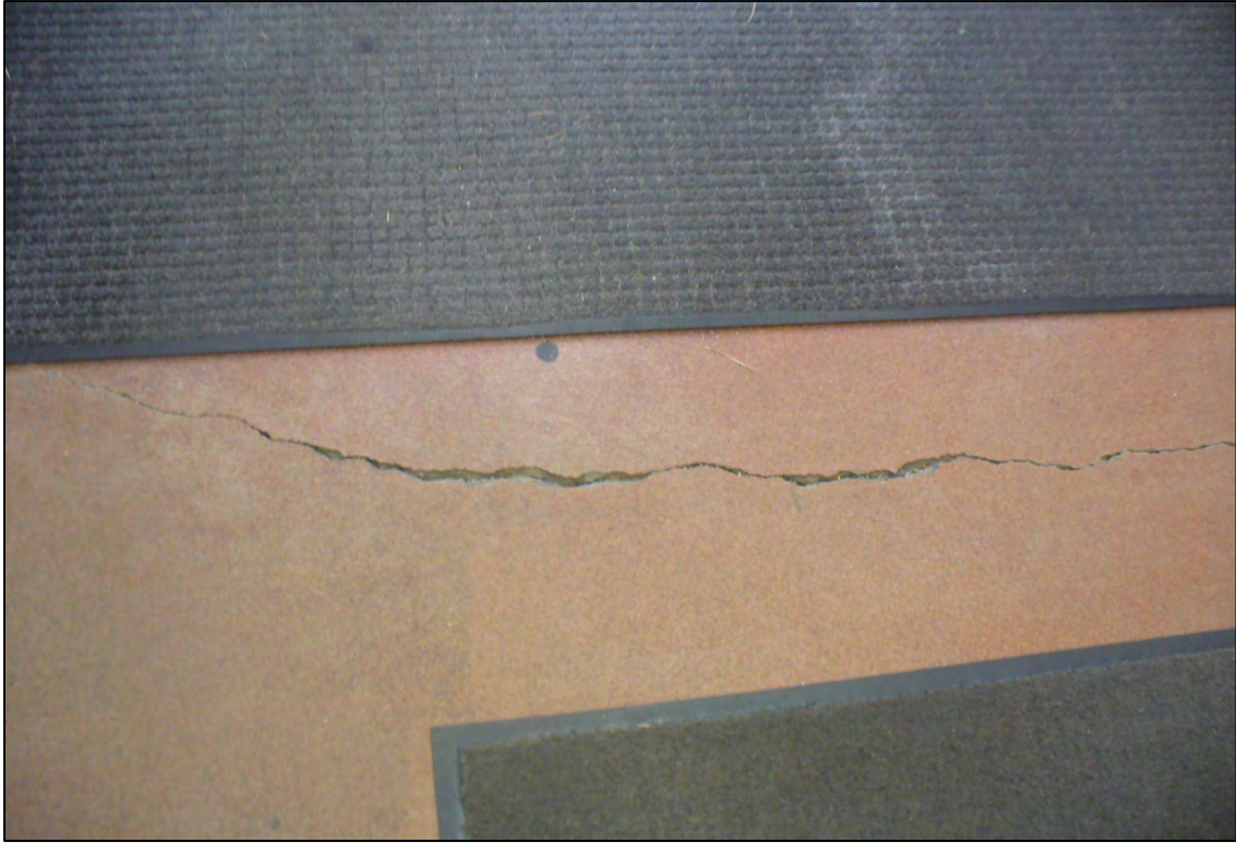
Floor cracks in concrete at vestibule on east entry at lower level.
