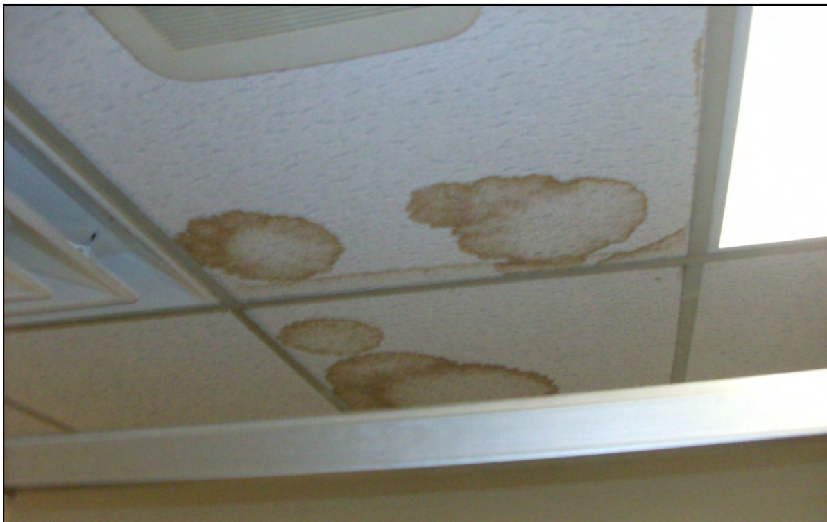
Stained ceiling tiles typical throughout building from pipe and/or roof leaks.
