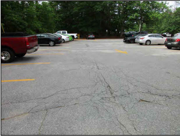
Cracked pavement on east side.
