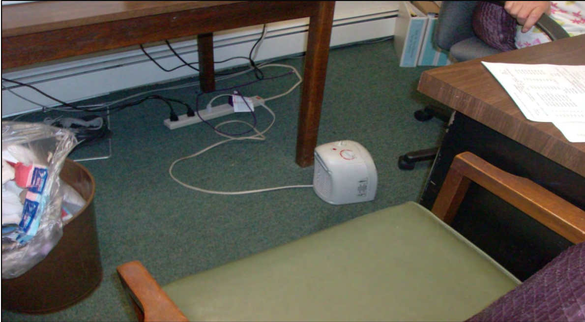
Lack of enough receptacles results in power strips and circuit overloads.
