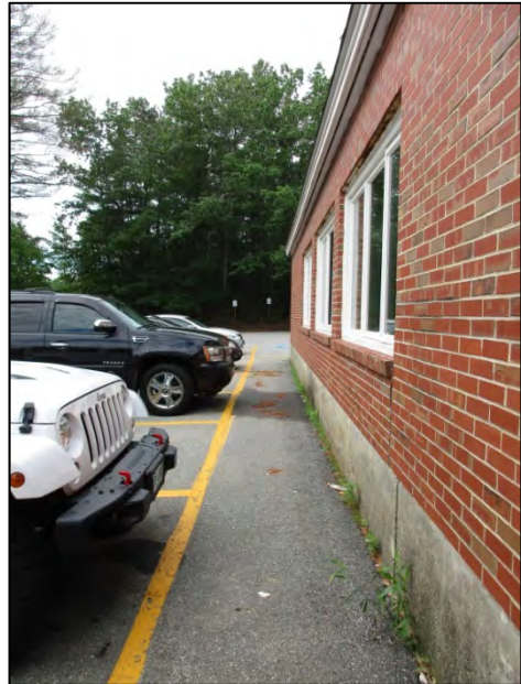
Pavement at face of foundation on east side. Note absence of roof gutter. Potential location for stone drip edge with underdrain. Installation of a guardrail or parking bumpers can help protect the building from vehicle impacts.
