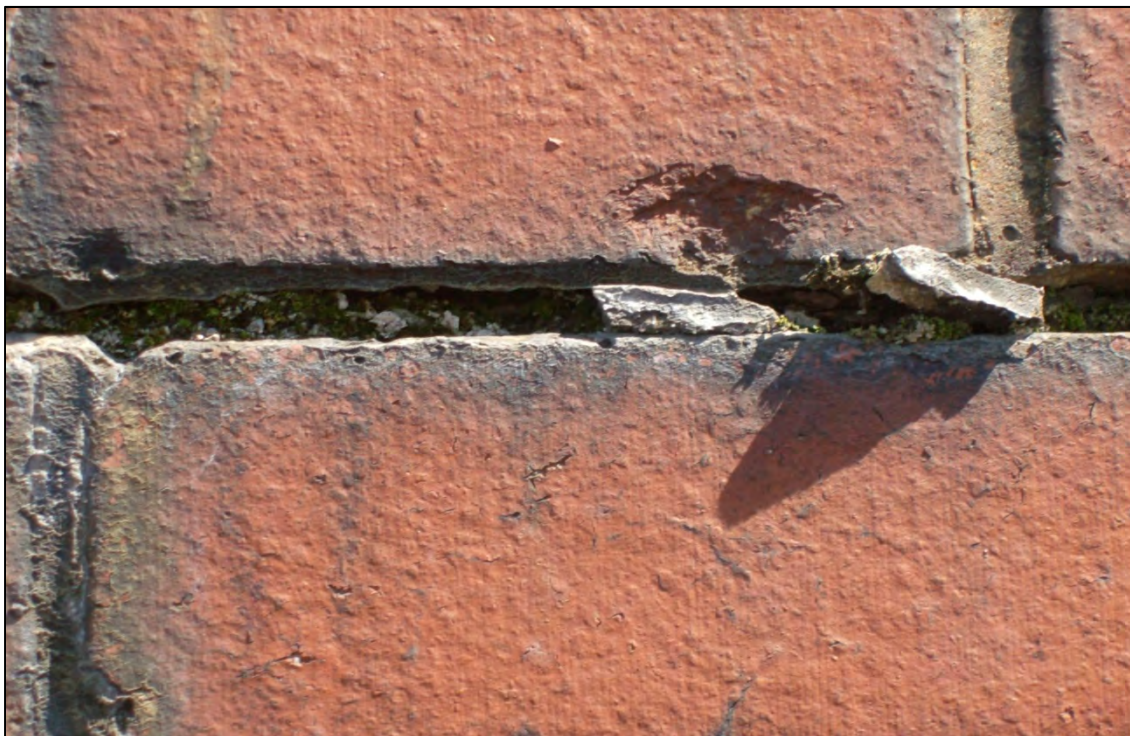
Repointing needed at brick chimney.
