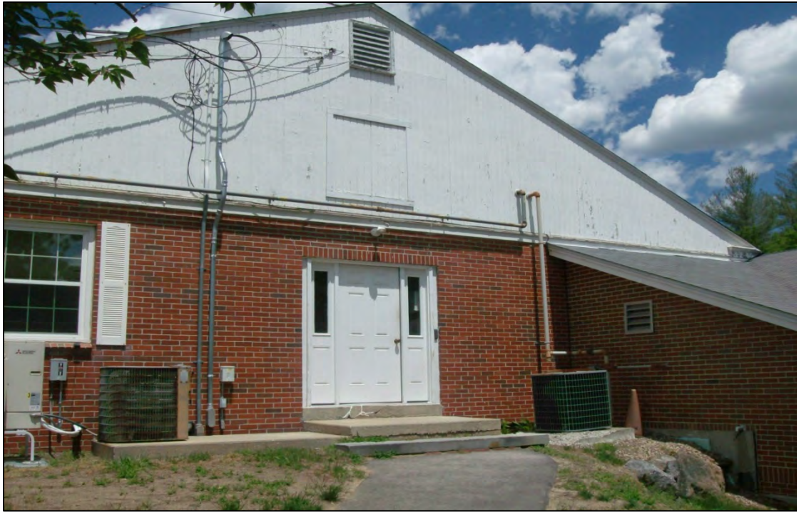
Peeling paint on gable end. Also note deteriorated compressor pad and cracked door sill.
