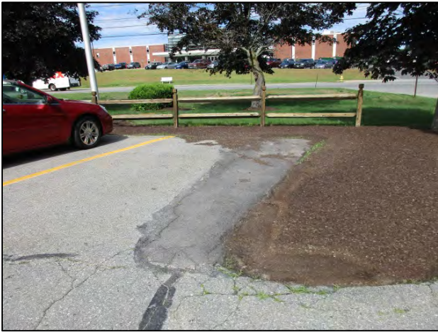
Drainage concern at the west side parking lot. Note evidence of ponding and the pavement repairs.
