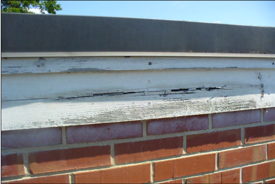
Rotted fascia on high roof over stairwell.
