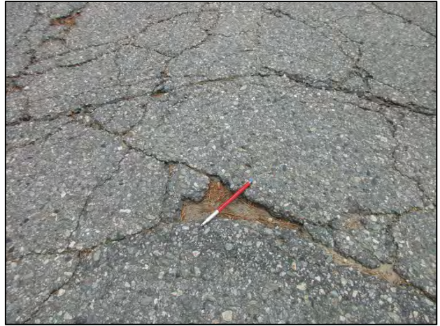
Enlarged detail of pavement cracking on east side.
