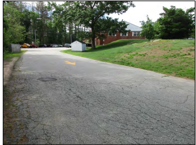
Fatigue cracking at exit driveway. Note sparse cover on vegetated slope adjacent to pavement.
