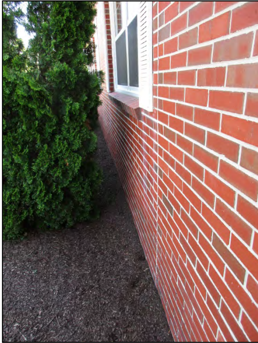
West face of building. Install stone drip edge
