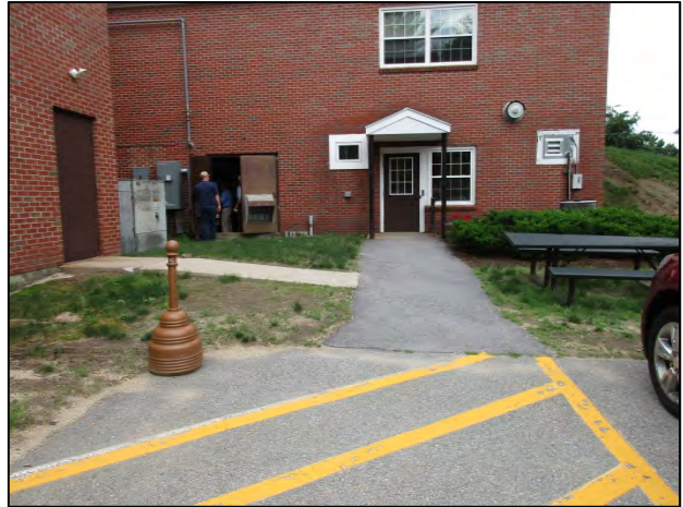
Sidewalks requiring ADA compliant railings.
