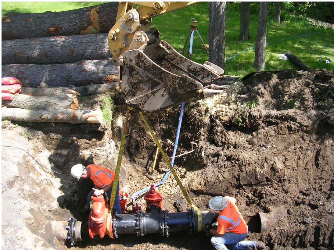
Installation of watermain
