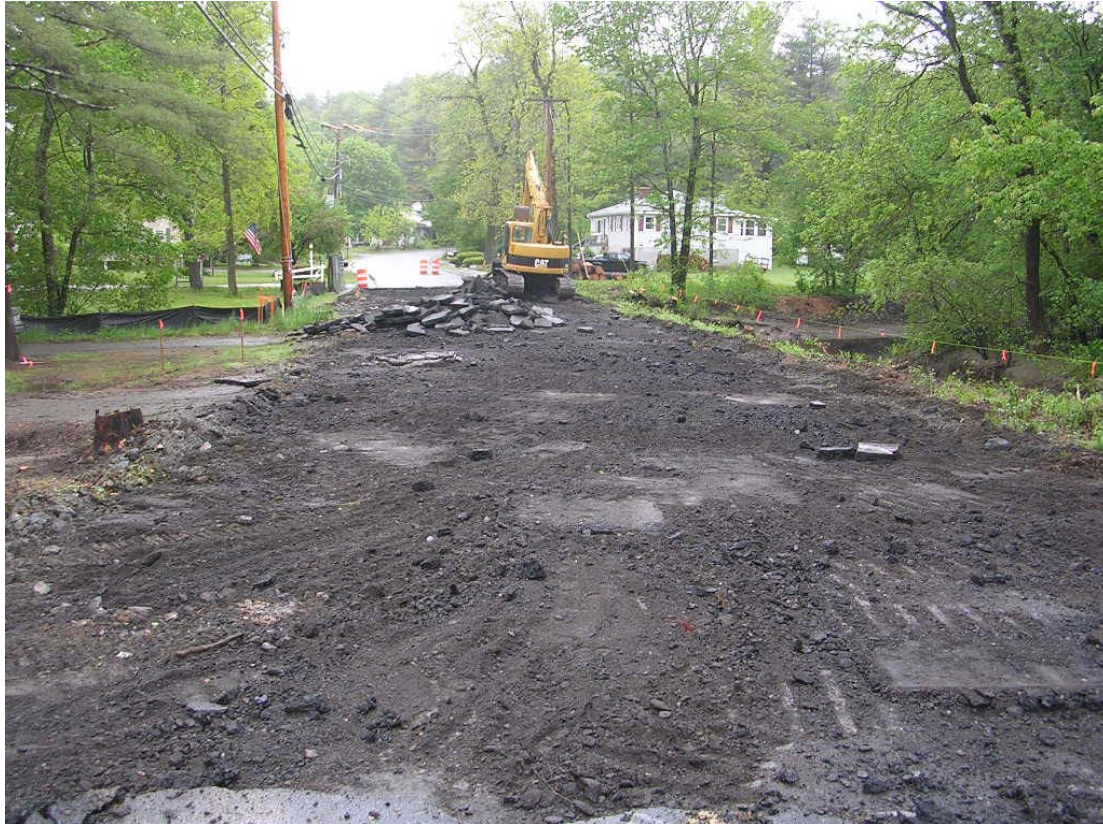
Excavation of existing pavement
