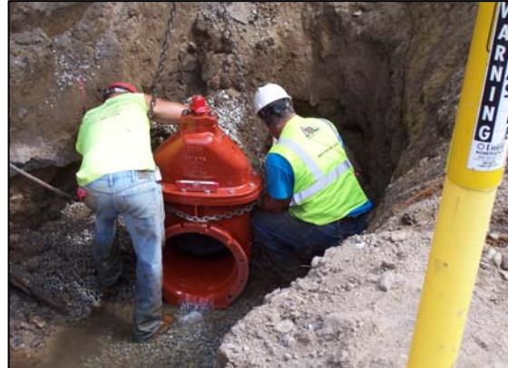
**Week 7.** The contractor was also working on excavation for the water main connection to the existing 16" water main. New gate valves and fittings were installed at each end to reconnect to the existing main.
