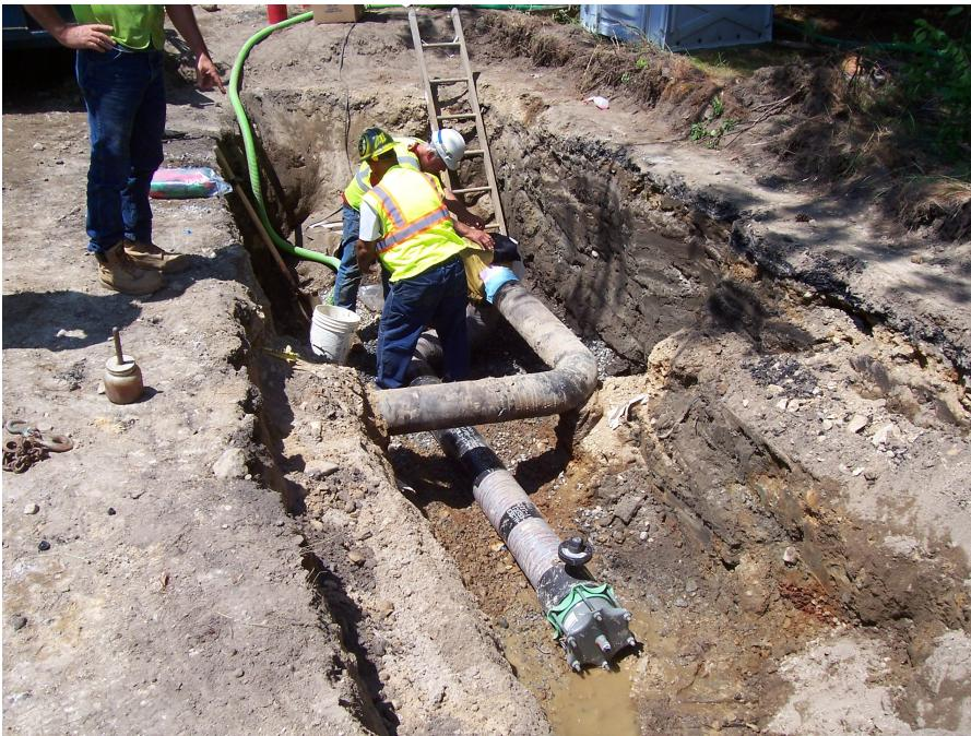
The Contractor also began of the Water Diversion system. Sand bag placement, excavation and pipe installation were underway. A temporary support for the gas line was constructed.
