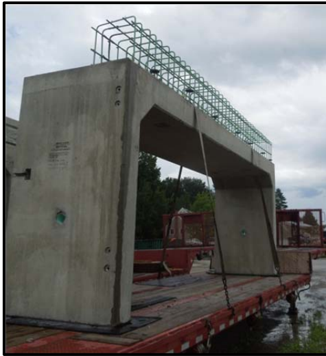
Rigid Frame Box Section after casting.
