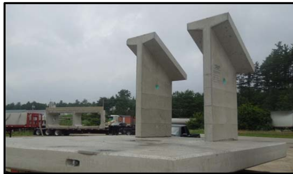
Wingwall section after casting.
