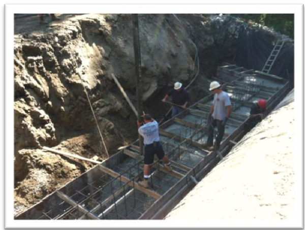
Concrete Placement at East Footing
