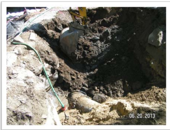
Excavation for the 24" water transmission line
