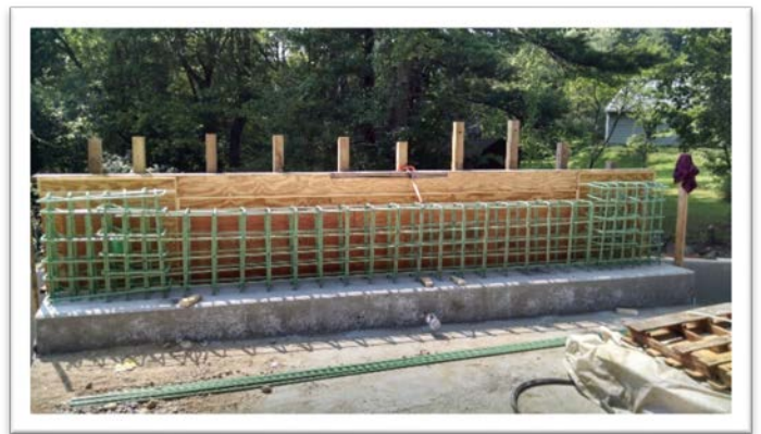
Bridge Rail Rebar
