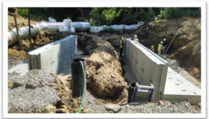
Bridge Footing and Stem Walls Installed
