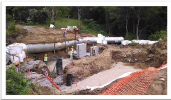
Installation of North Footing and Stem Wall
