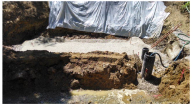
Structural Fill for South Footing
