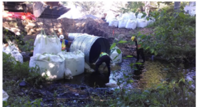
Installation of Diversion Pipe (Upstream)
