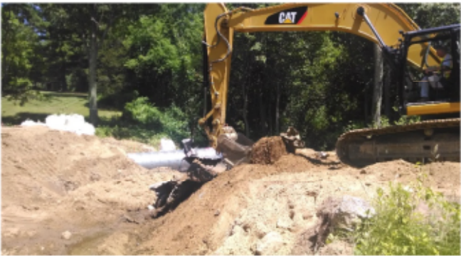
Removal of Culvert
