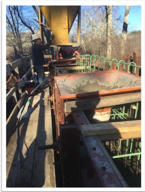
Pouring Concrete for the New East Abutment Wall Looking North/Upstream
