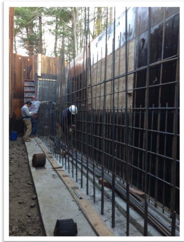
Tying Reinforcing Steel for the New West Abutment Wall - Looking South/Downstream
