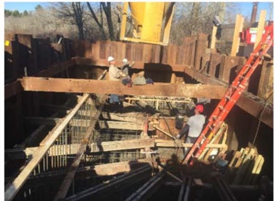
Placing East Abutment Footing Looking Upstream/North
