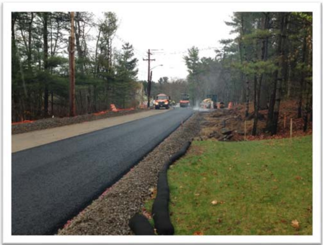
Paving Base Asphalt Course – Looking East Towards the Bridge
