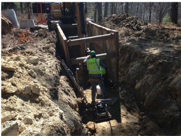
Ledge Removal for Installation of New Drain Pipes and Structures at Town Farm Rd - Looking South
