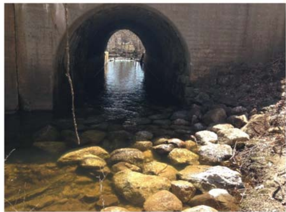
Scour Hole Filled with Riprap – Looking Downstream/East
