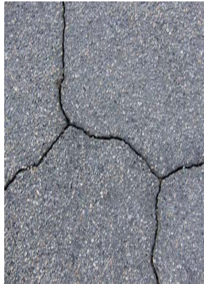
Block Cracking
