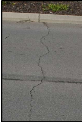
Transverse & Reflective Cracking
