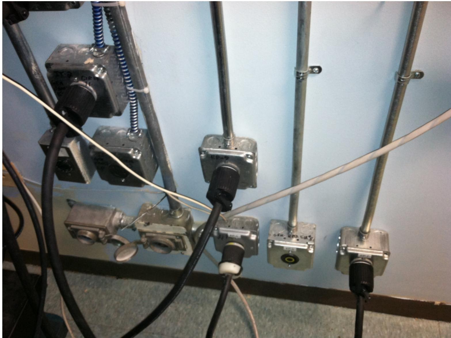
EXISTING POWER OUTLETS SUPPORTING THE SERVERS, TO BE REPLACED WITH NEW AND ORGANIZED ON THIS SAME WALL. IN ADDITION, PROVIDE THREE (3) QUAD OUTLETS ALONG THIS WALL FOR STANDARD POWER NEEDS.
