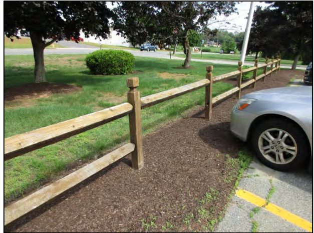
Replace fence rail.
