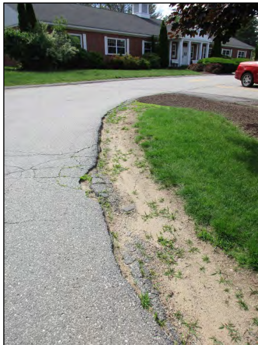
Poor grass cover and erosion along edge of pavement.
