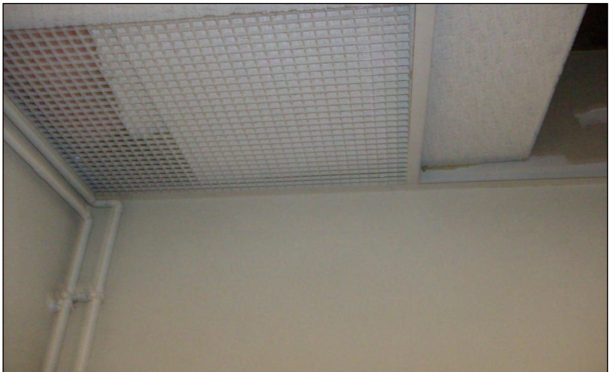
Open ceiling grate in east side bathroom to let warm air above ceiling so pipes don't freeze.
