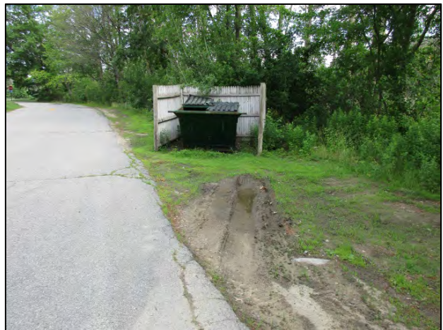
Vehicle approach to dumpster. Gravel surface susceptible to rutting. Note gravel surface beneath dumpster.
