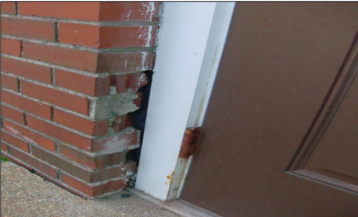
Large gaps left behind brick façade when door frame was cut in and installed.
