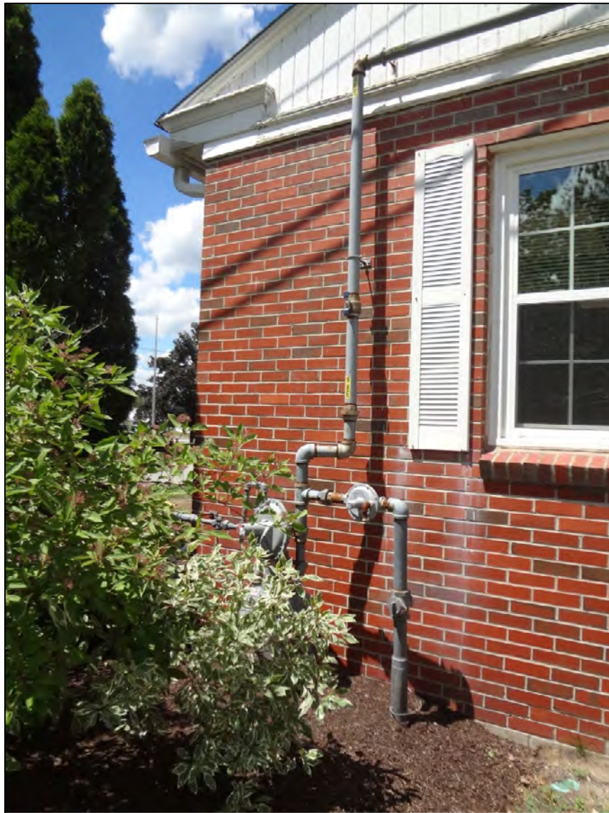
Gas regulator close to window.
