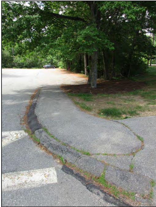
Failing sidewalk pavement and bituminous curbing. Paint a white or yellow stripe along the top edge of curb.
