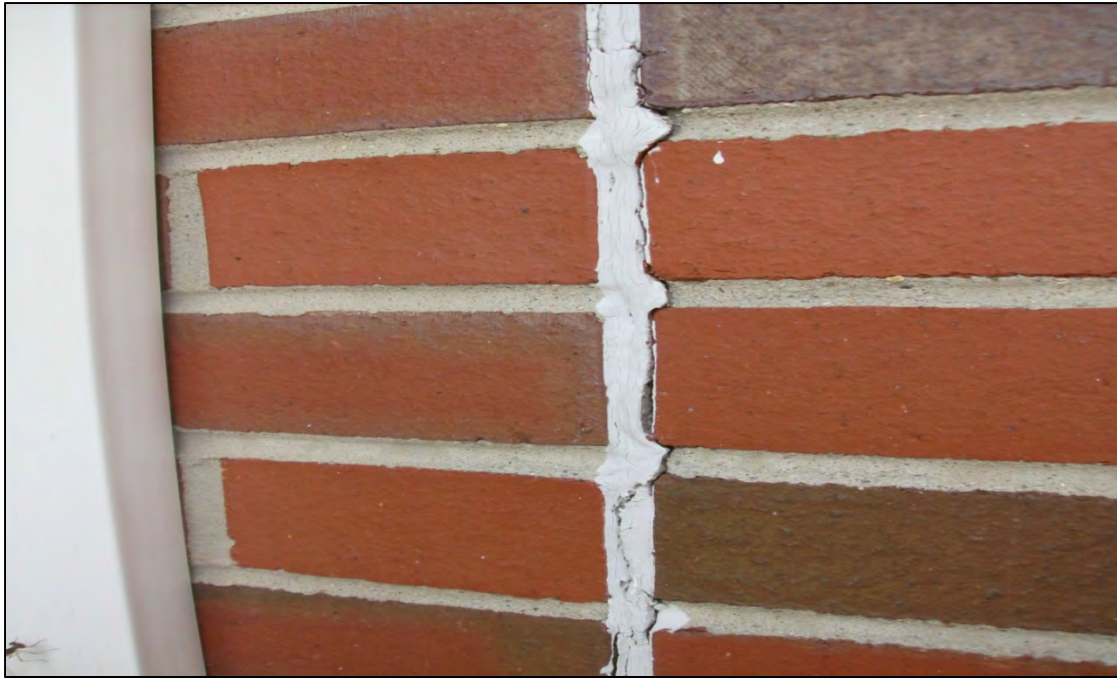
Failed control joint sealant.
