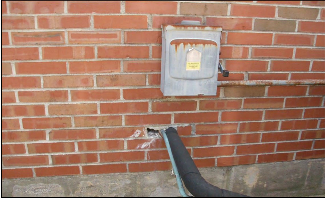
Open hole in brick face allows air and moisture infiltration, as well as access for insects and rodents.
