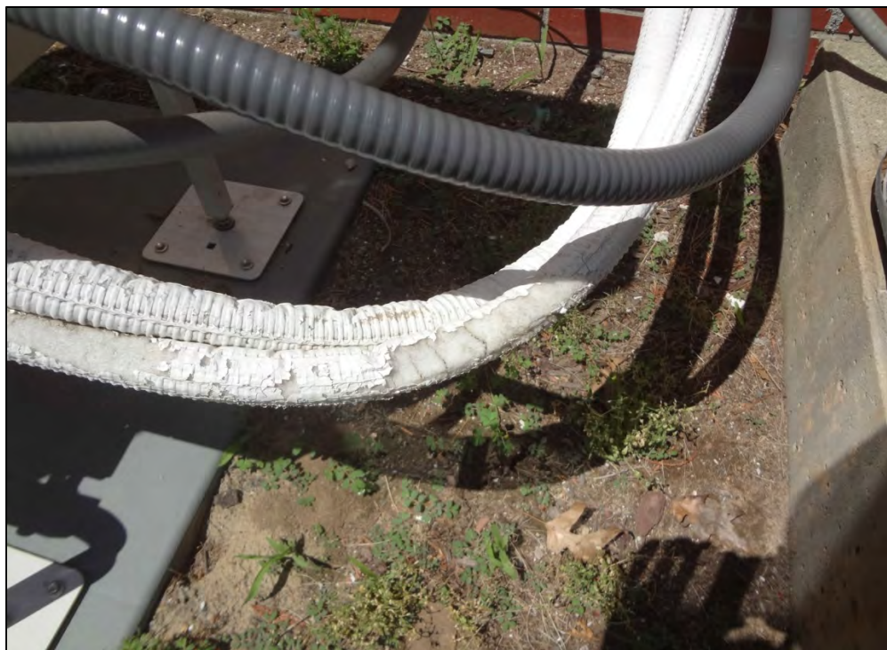
Insulation on cooling lines needing replacement.
