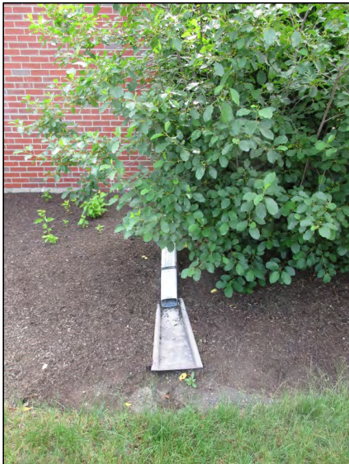
Gutter outlet at southwest corner of building. Tie into an underground piping system to eliminate direct discharge.
