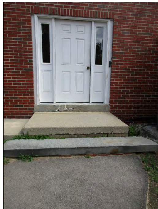
Stairs at southwest entrance. Replacement required for compliance with ADA. Note absence of handrails.
