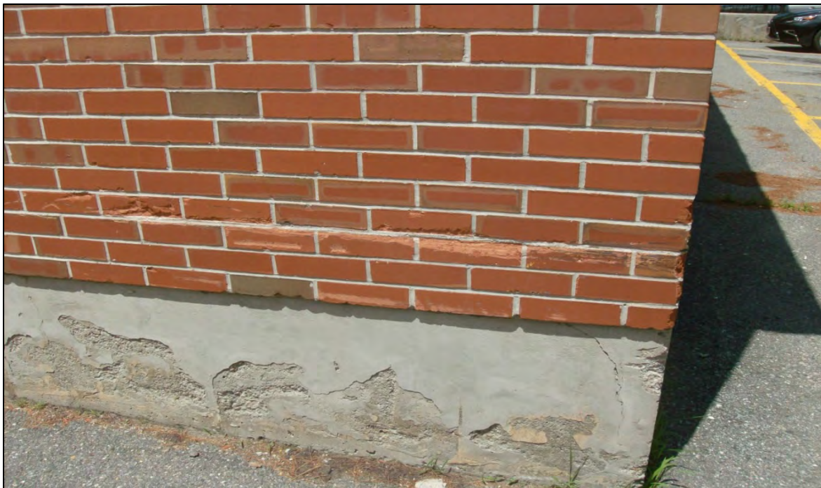
Damaged and cracked concrete and damaged brick at southeast corner.
