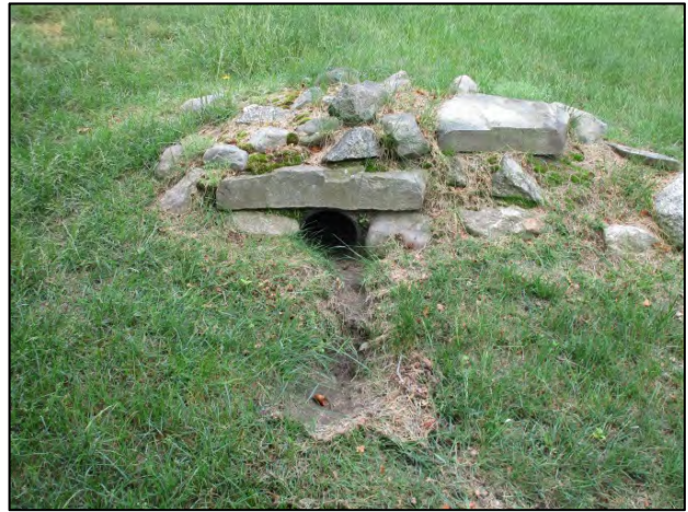
6-inch roof drain outfall on the north side.
