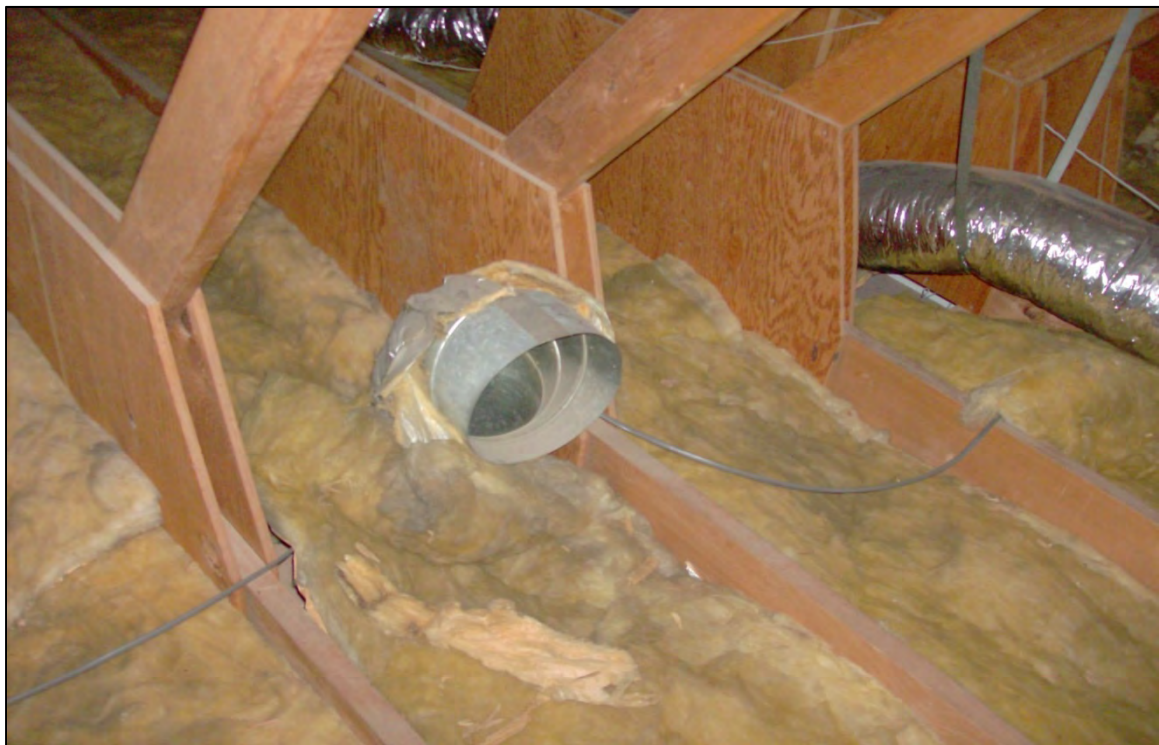
Insulation in attic space over original building, plus old abandoned ductwork open to the space.
