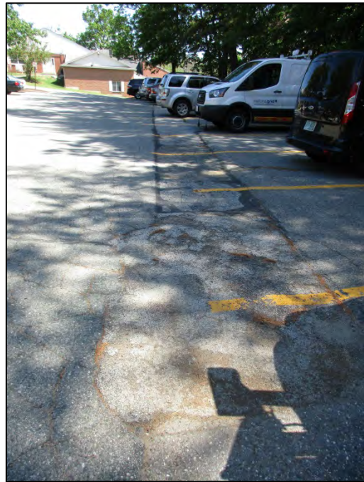
Pavement deterioration at south side parking lot.
