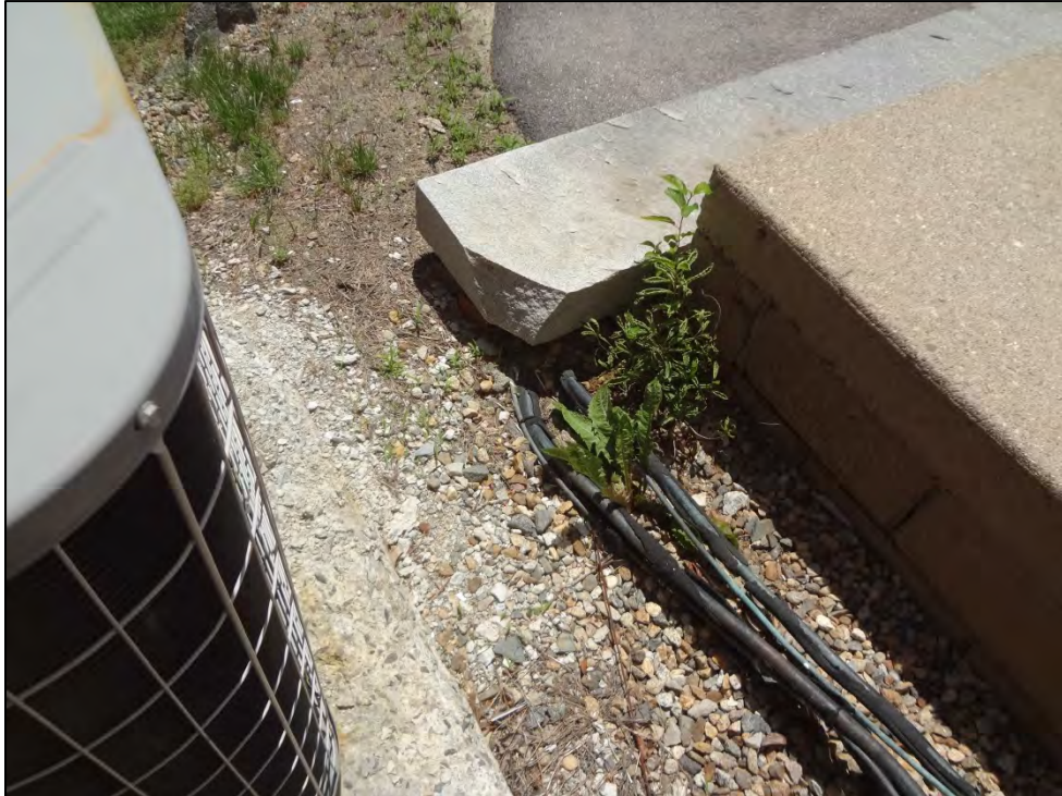
Refrigerant piping under stair and bad insulation.
