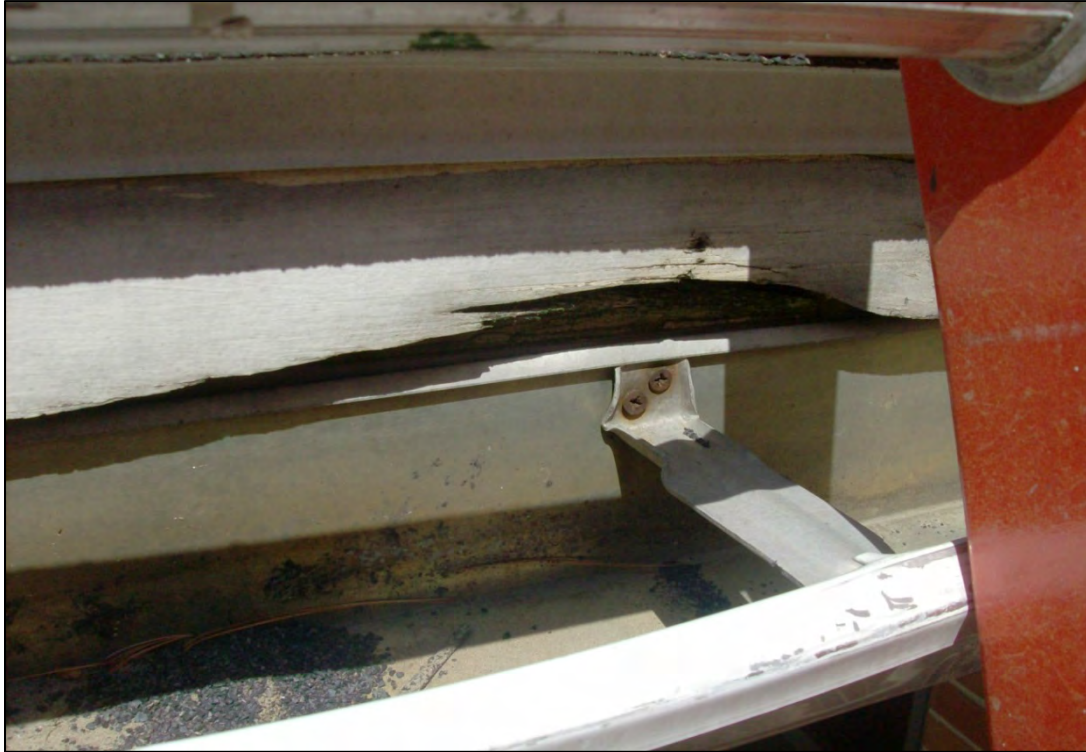
Rotted fascia board on east side.
