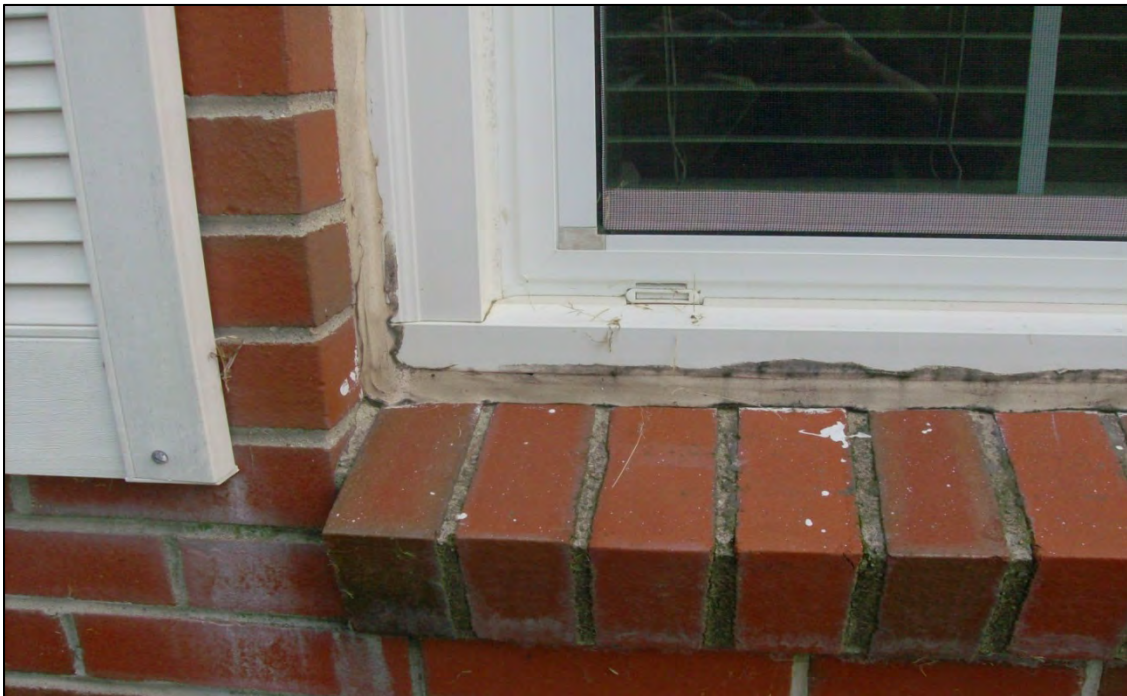
Sealant around window needs replacement.
