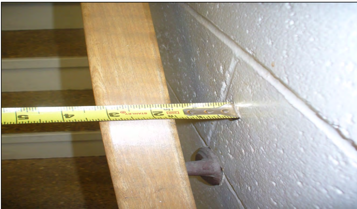
Non-compliant stair rail on communication stair between upper and lower levels.
