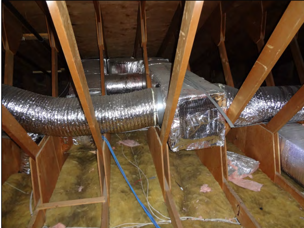
Attic ducts excess flex and poor insulation.
