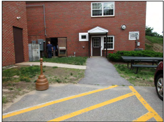
Sidewalks requiring ADA compliant railings.
