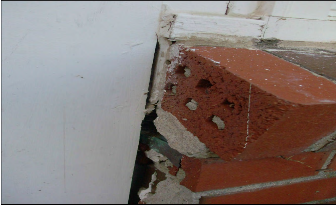
Doorway cut into wall at finance department left large gaps between trim and brick façade.
