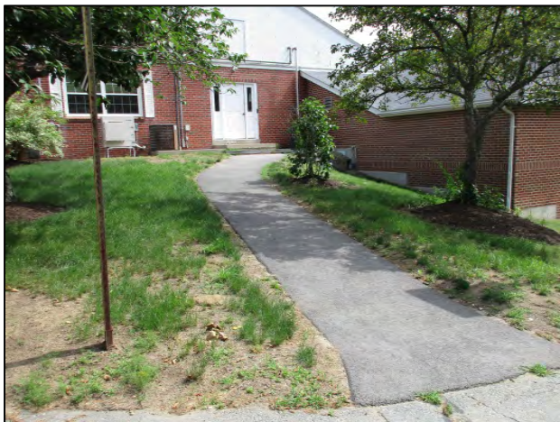
Sidewalk with 10% slope; no railings or landings.
