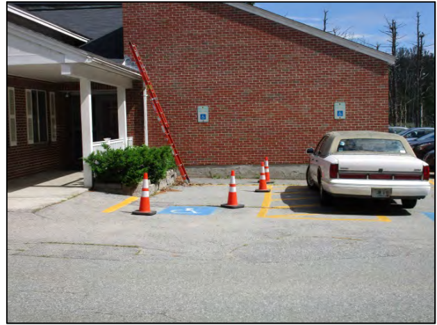
Accessible spaces adjacent to south side of Town Hall. No 'Van Accessible' signage and the slope up to the concrete sidewalk is excessive.
