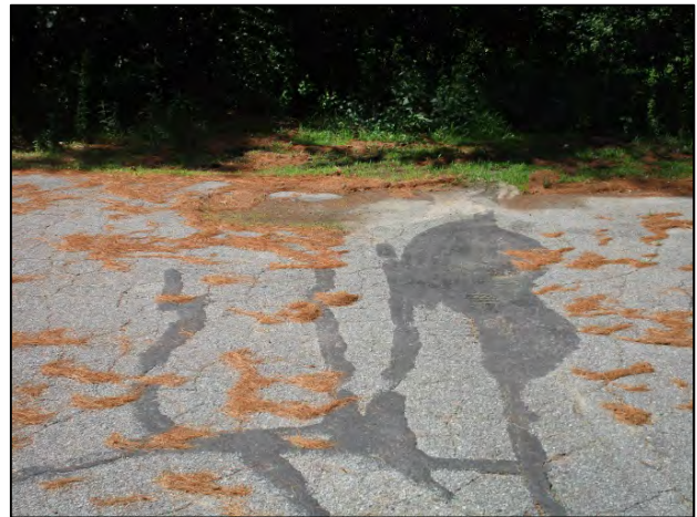
Pavement deterioration and evidence of past repairs where south side parking lot drainage runs off the asphalt and into the wooded area between Town Hall and the Courthouse site.
