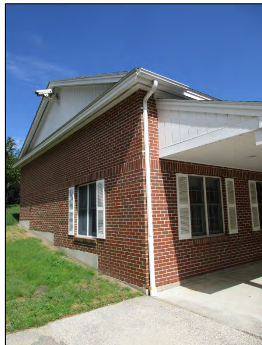
Roof gutter on the south side of the building connected to an underground system. Underground system likely crosses east parking lot and discharges in wooded swale on east side of property.
