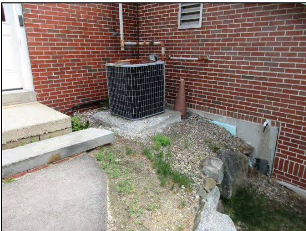
Stone retaining wall requires a guardrail and the concrete pad beneath the mechanical unit is deteriorating.
