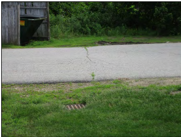
Drop inlet along exit driveway. Note pavement crack above pipe.
