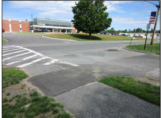
Entrance driveway at intersection with Geremonty Drive. Cracking, trench repairs. Note undersized sign.
