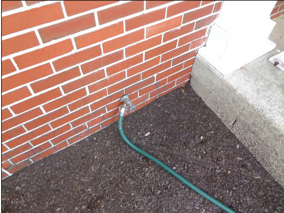
Hose bibb lacks vacuum breaker.
