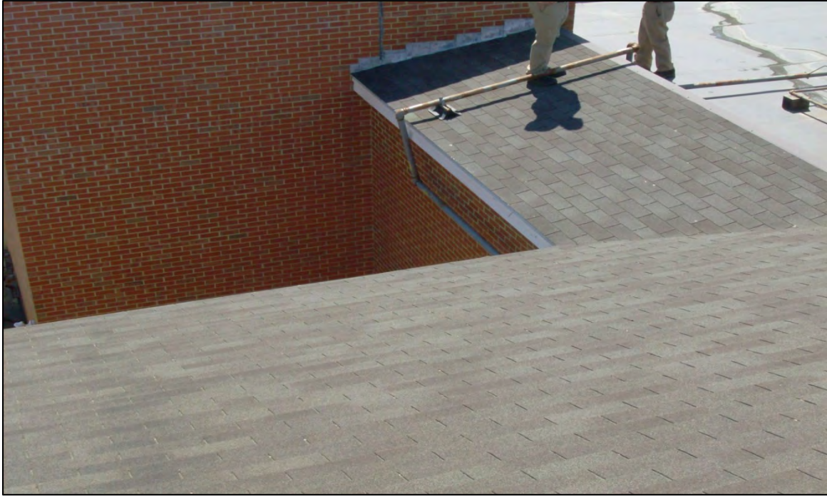
Exposed gas line to boiler room runs over roof and across north wall.
