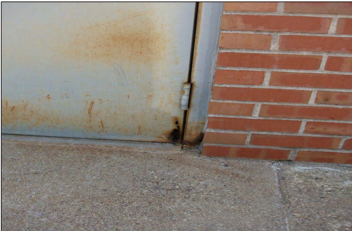
Rusted door and frame at mechanical room at northeast corner.
