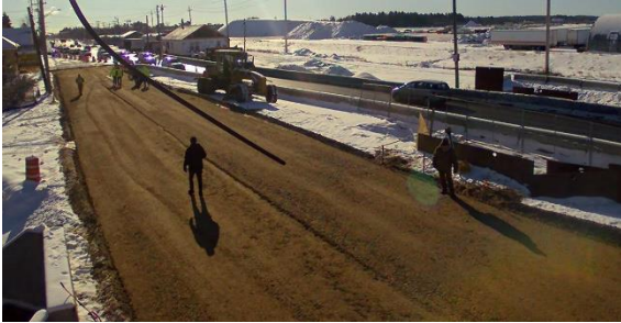
Gravel Installation on Bridge Phase 1
