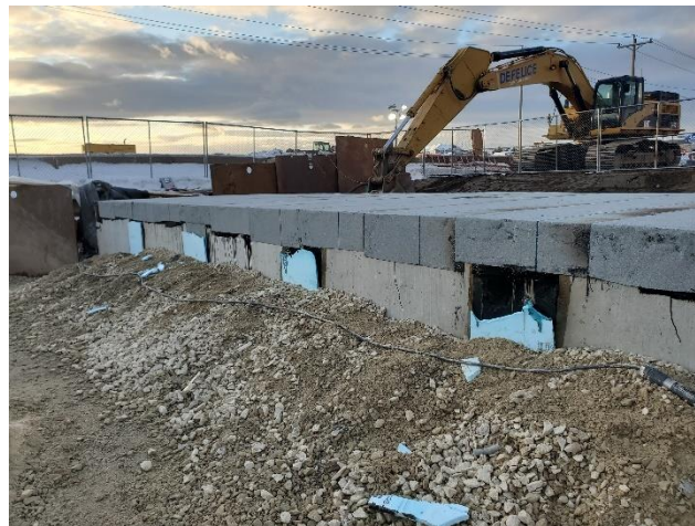
Water protection Membrane Installation
