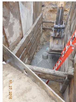
Sewer Service Chimney installation
