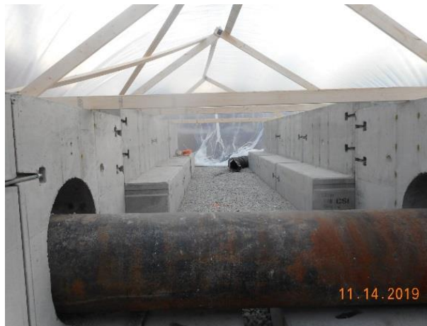
Temperature controlled Tent for grouting
