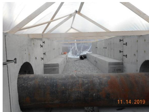
Heated tent setup for concrete and grout curing
