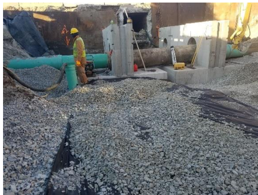
Sewer reinstalled within new footing
