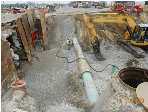
Sewer Preparation work for Bridge Footings
