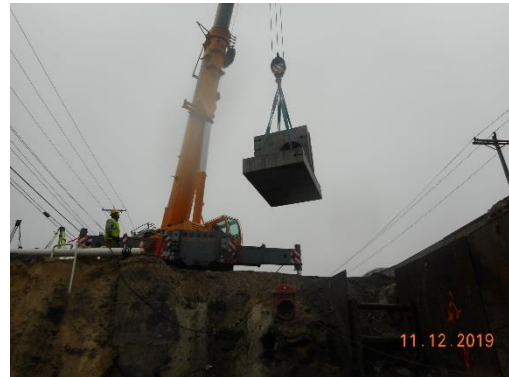
Beginning of Bridge footing installation
