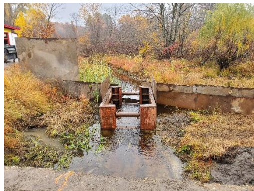
Stream Bypass Preparation for Bridge Construction
