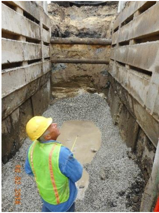
Sewer Trench Bedding Installation
