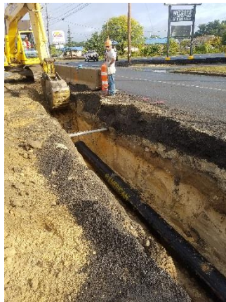
New Water Main Installation
