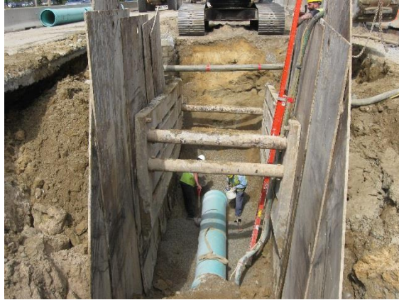
Sewer Main Installation
