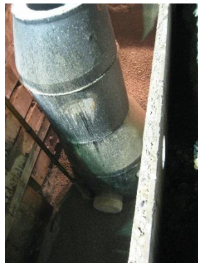
New Sewer Manhole
