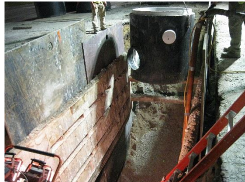
Sewer Manhole Installation
