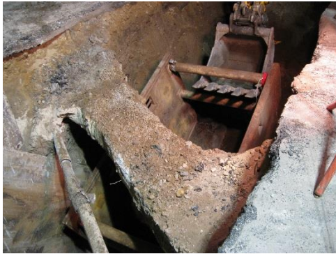
Sewer Trench Box Installation
