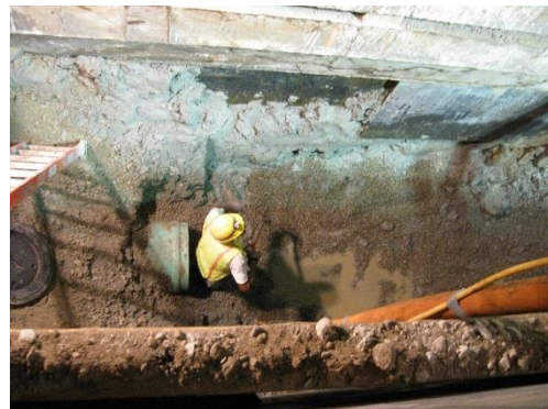
New Sewer Main Installation
