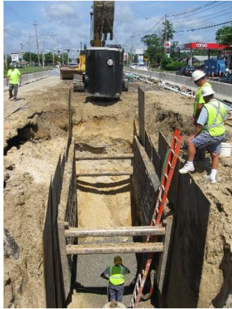
Sewer Manhole Installation
