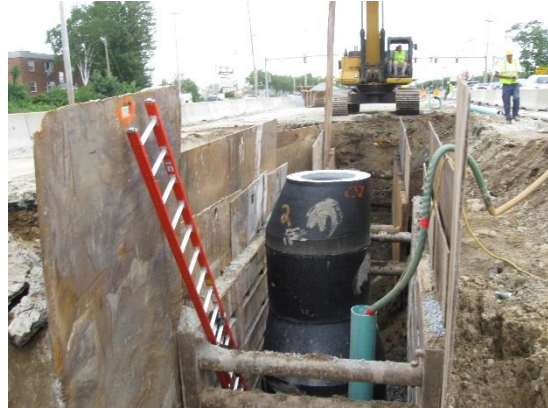
Sewer Manhole Installation
