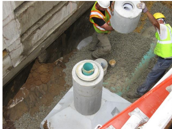
Sewer Service Chimney Installation
