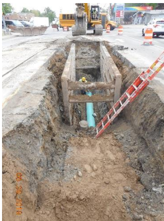
Sewer Pipe Installation
