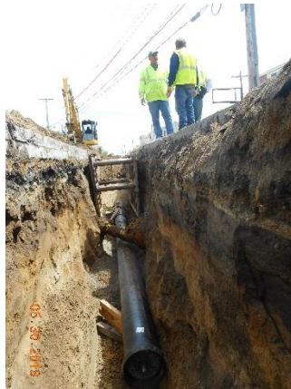
Water Main Installation
