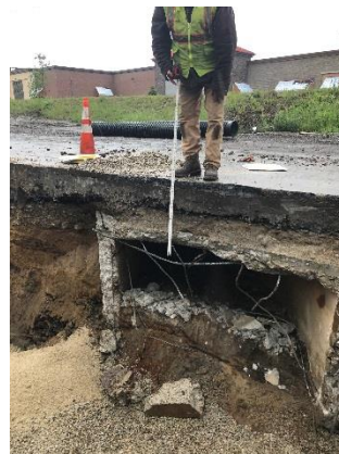
Test Pit Investigation at Culvert
